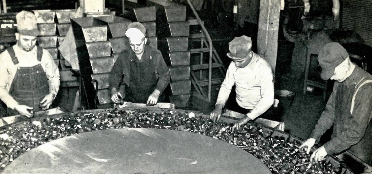
Castings are sorted for grinding at this slowly revolving table, which makes a complete revolution every four minutes. In that time it is capable of taking a full load of 3,600 pounds of castings from the Ransohoff "water rattler," a machine that washes and polishes the castings. Sorters at the table include, from left to right: Fayne Marohl, Floyd Durbin, George Shotten and George A. Hill.
