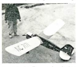
it carried a pilot. The gas tank carries three ounces of gas, which will run the motor for thirty-six minutes, and when the gas supply is exhausted the plane automatically goes into a glide and for every foot of altitude the plane will glide seven feet. It is designed so that it is inherently stable, that is, any upsetting forces will be automatically compensated.
