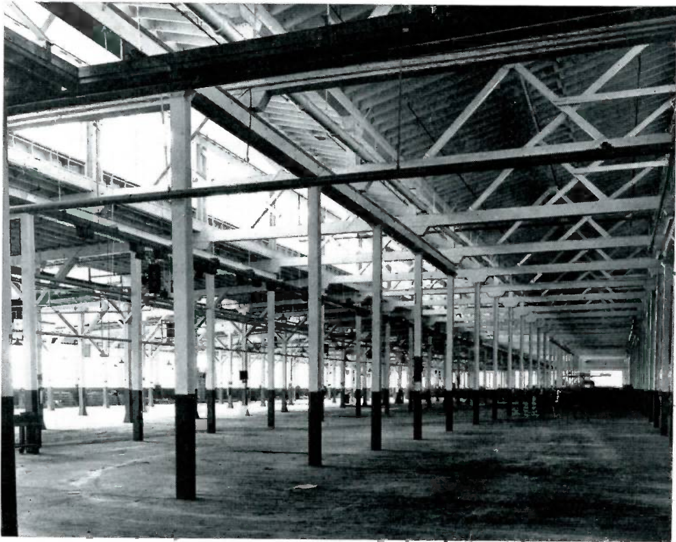
Interior view of the main building. The truck shown at the right indicates building's size.
