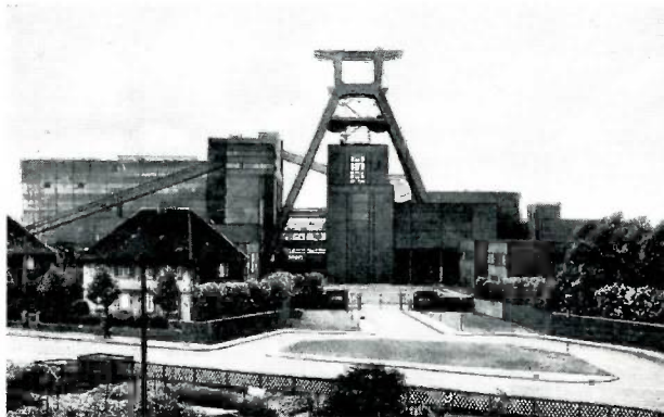
Shafts 1 and 2, Zollverein coal mine, Essen.
