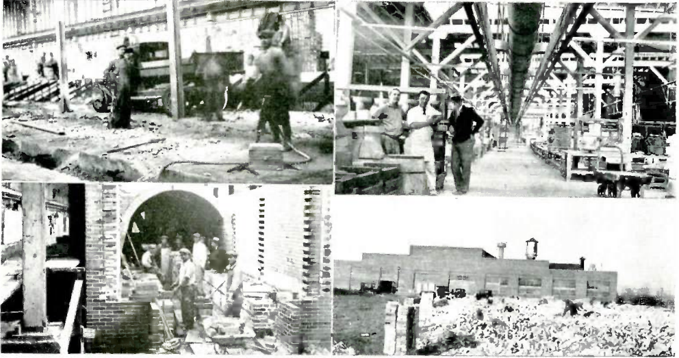
The past winter witnessed great activity at Plant 3. Upper left: Getting rid of old kiln and preparing for new; Upper right: In the casting shop, A. H. Culver, Wm. Burchell and J. A. Richardson in the foreground; Lower left: Building the new kiln; Lower right: Cleaning brick from old kiln.
