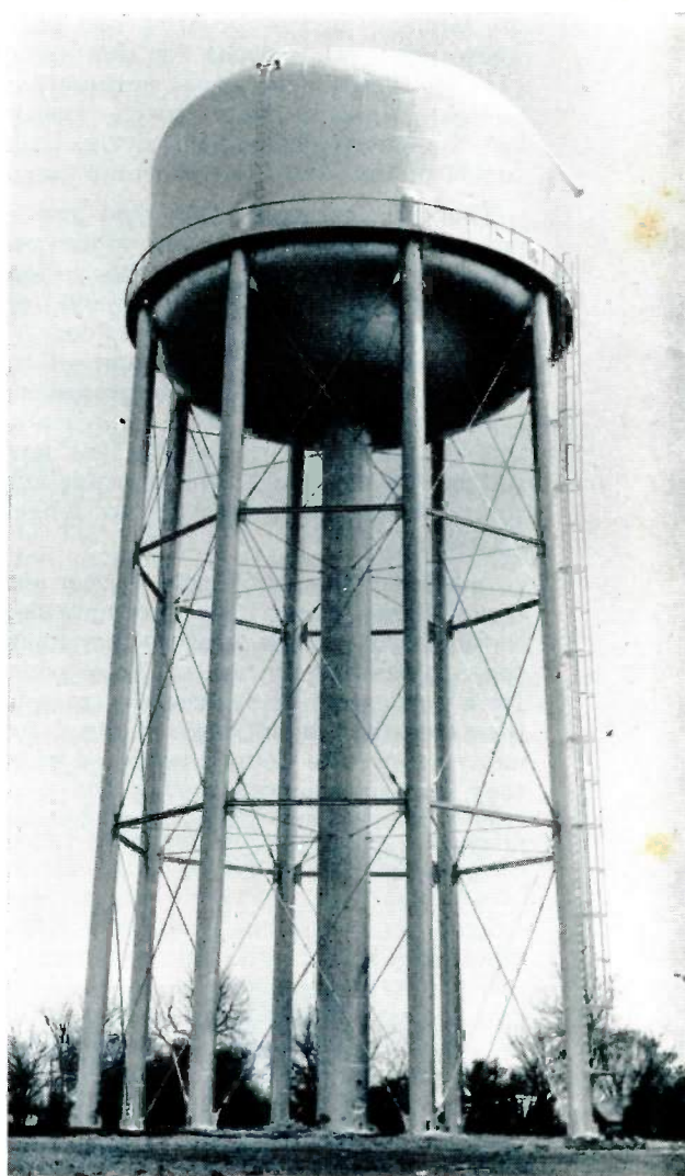
The new 500,000 gallon elevated tank which replaced a 100,000 gallon capacity standpipe is a part of initial improvements paid for by the city's $250,000 bond issue.
