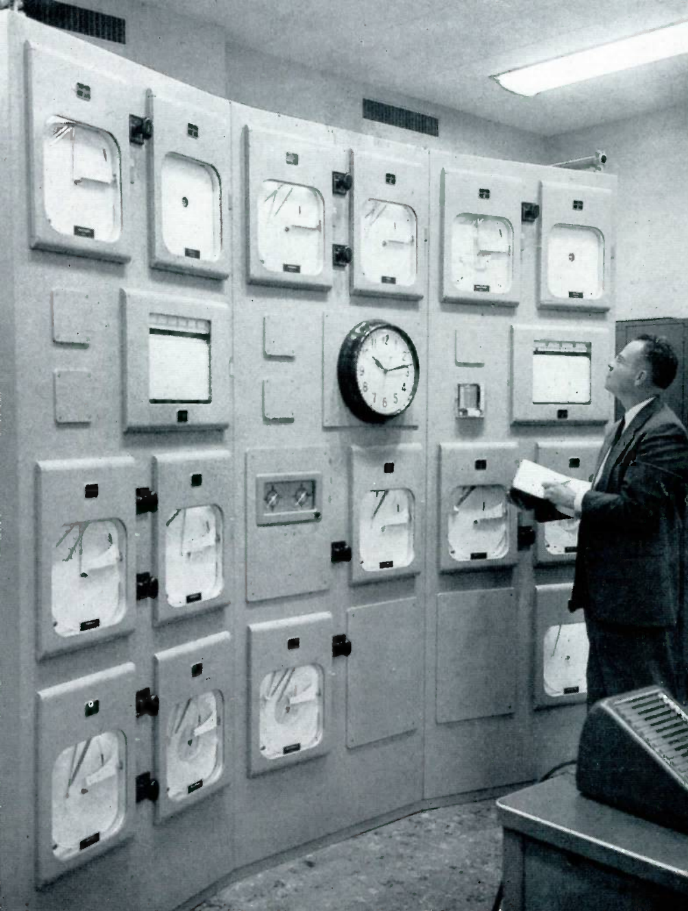
Illinois Power uses teletesting instruments in Decatur to measure the amount of gas purchased from four of their five pipeline suppliers. It has been praised as one of the most advanced systems of its kind in the country.
