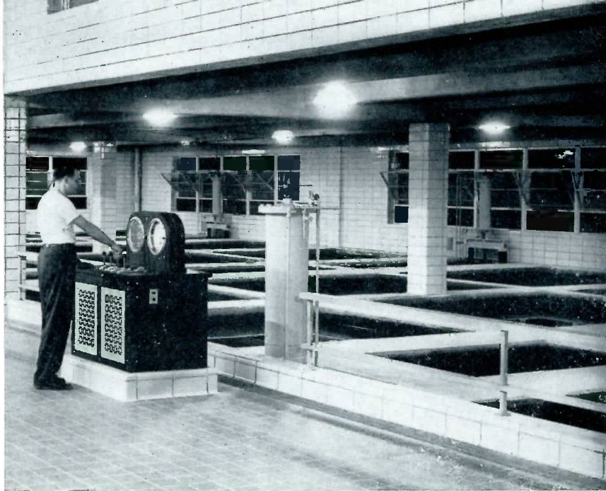
These are the new five million gallon capacity filters, located at the Oradell Purification Plant. This modern plant is capable of filtering 100 million gallons daily.
