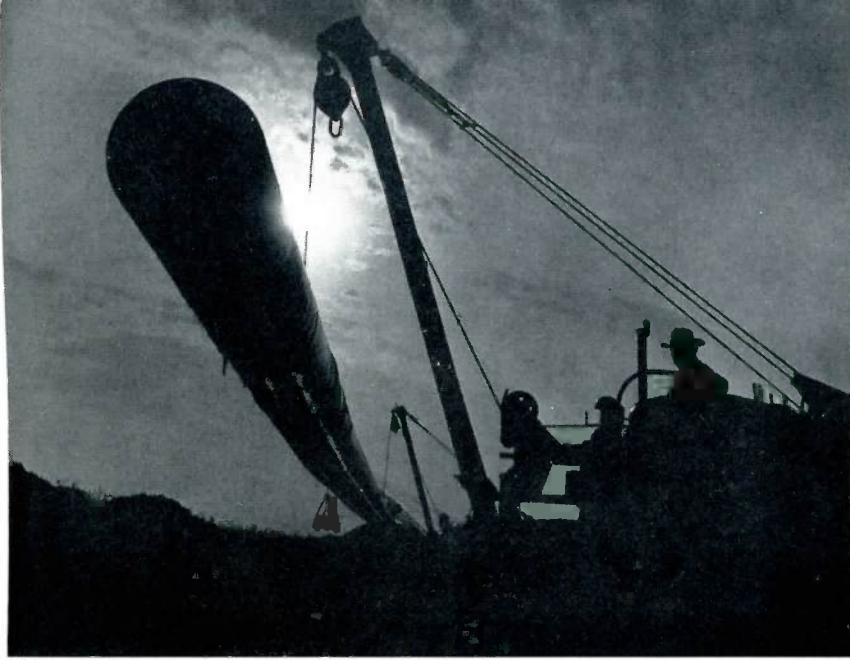
The work of Illinois Power crews is never done, as the utility constantly expands to meet the needs of population and industrial growth in the area which it serves.
