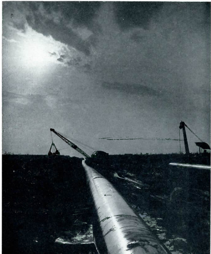
Mains stretch into the horizon in this dramatic night shot. Two thousand, three hundred and forty-eight miles of mains wind their way to sixty five communities in the state.
