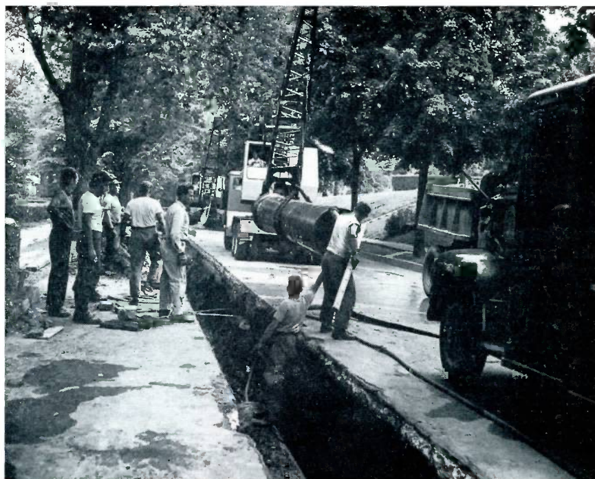
A Hackensack Water Company crew works on a transmission main installation project to serve the expanding territory in northern New Jersey.
