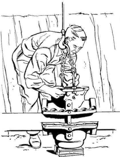
1. Bolt sleeve halves to main and calk end joints.
