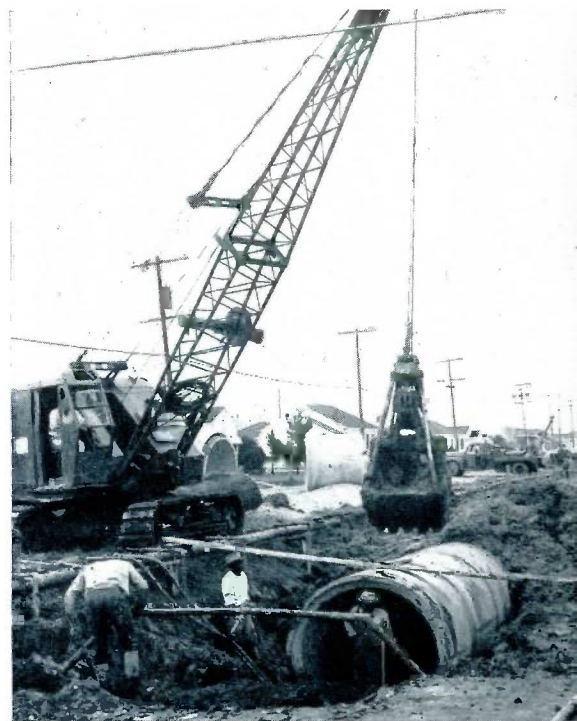
This photo shows the covering process on the St. Roch Canal.
