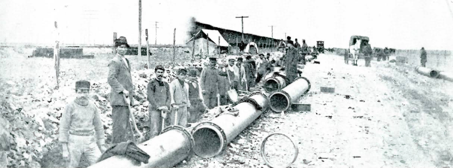
Even the plodding machines of 1909 were a big improvement over the use of shovels and back muscles. Here workmen are shown laying Lone Star's first long distance
