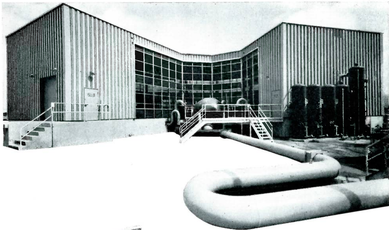
Most of the main features of the new Long Beach compressor plant are shown above. It shows the plant's grouping around the gas suction sphere, the donut shaped ring header and the inlet pipe from the holder. The lower photo shows the gas holder piston dome size in relationship to a workman.
