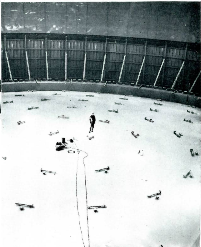
Most of the main features of the new Long Beach compressor plant are shown above. It shows the plant's grouping around the gas suction sphere, the donut shaped ring header and the inlet pipe from the holder. The lower photo shows the gas holder piston dome size in relationship to a workman.
