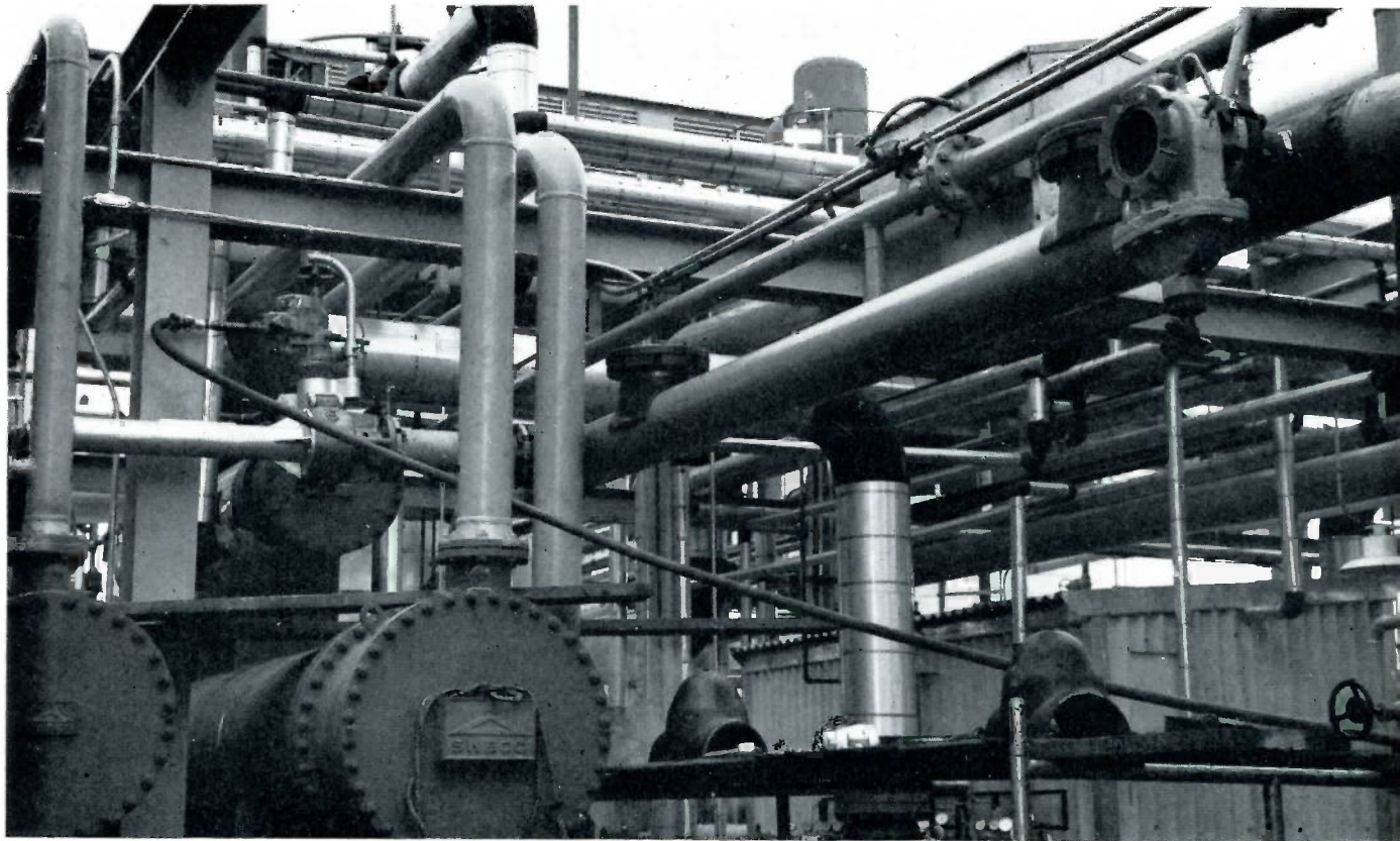
Almost hidden in this maize of pipes is the Mueller C1-36 drilling machine which is making a lateral cut for a four-inch by-pass line. The top sections of the fittings are shown in position on the pipe and mark the section of the pipe that was to be isolated. The gate valve at the right is inverted because of space limitations.
