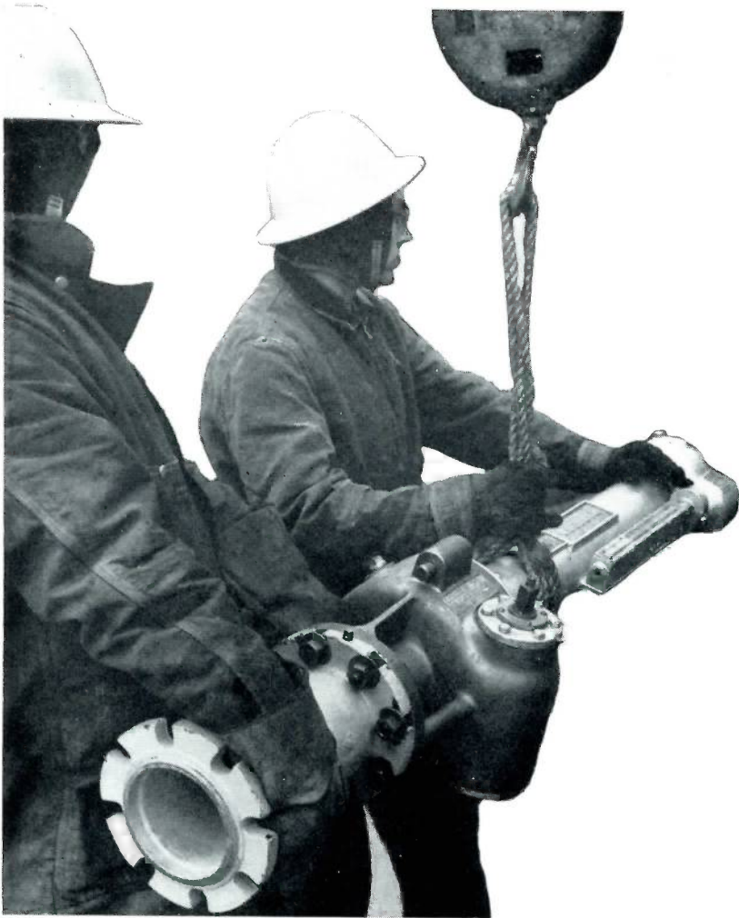
Workmen are shown guiding the Mueller drilling machine and its adapter into position prior to making a four-inch cut for the by-pass line.
