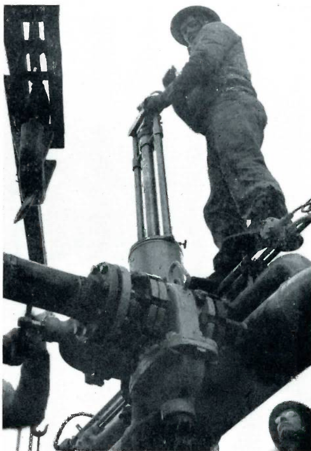
After the separator was welded in the line, the workman (above) withdraws the stopper preparatory to completing the job. At the right the completion plug and its inserting machine are being lowered into position. Sticking out on the left of the body of the completion machine is a special purging connection.
