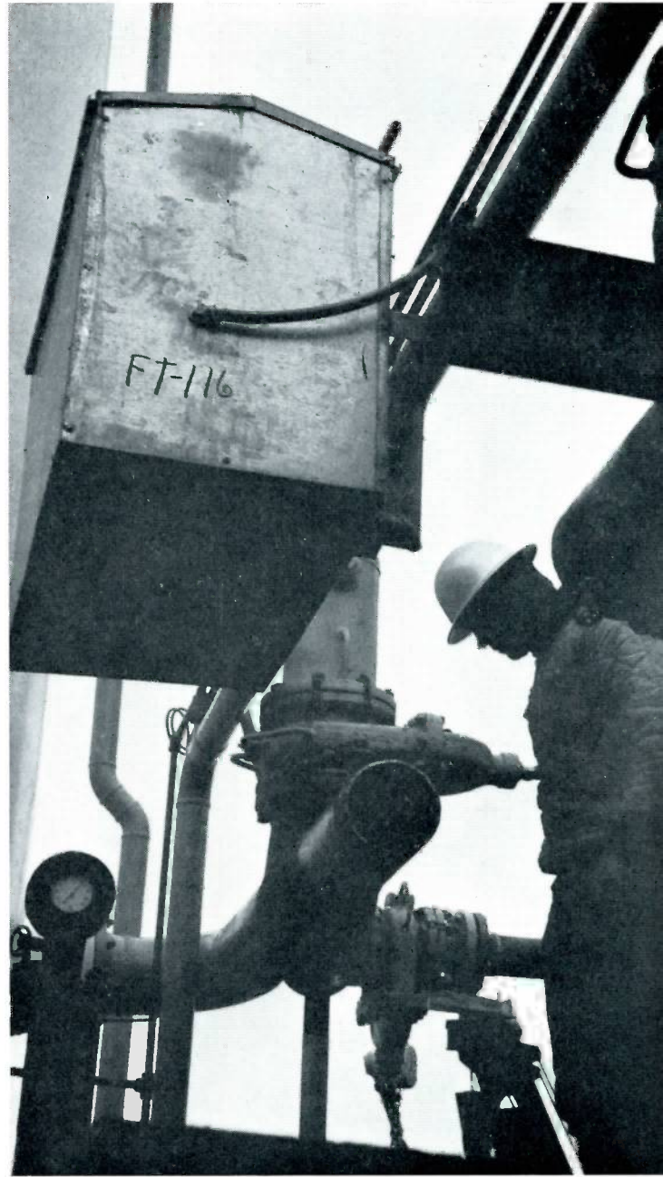
A four-foot section of pipe has been cut from the line but the plant continues to operate without interruption as the Mueller line stopping machines divert the flow of hydrogen gas through the by-pass line.
