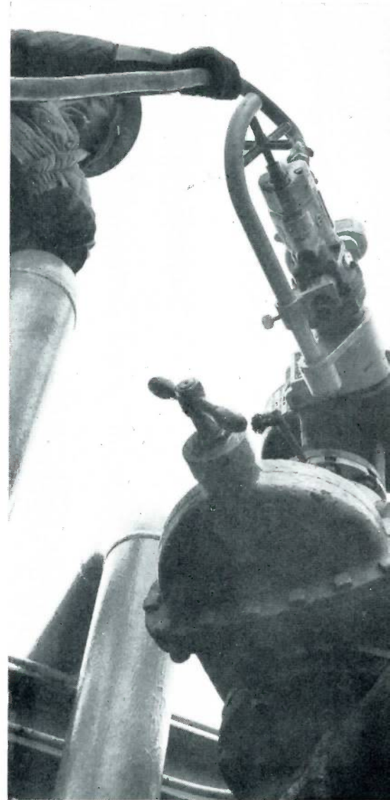
The machine is now in place and the machine's shell cutter begins its descent through the eight-inch pipe which is carrying hydrogen at about 100 psi.
