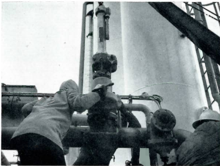
Mueller Project Engineer Lynn D. Edwards (left) closely observes the machine being bolted to the gate valve prior to making the first eight-inch cut.
