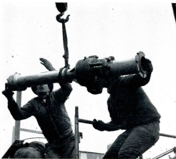
The machine is now in the air and is being swung into position (left). In the photo at the right, the C1-36 ma-
