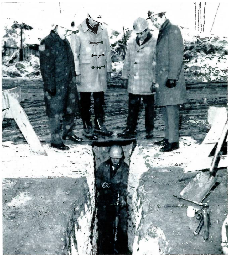
Checking a tap being made with a Mueller D-4 Machine at Expo 67 are, from left, Mueller, Limited Sales Representative Art Hutchingame; G. F. Proulx, Chief Inspector for Quebec Natural Gas Company; M. Perron, Chief Inspector for the gas distribution system at Expo 67, and Mueller, Limited Sales Representative Wilf St. Cyr.
