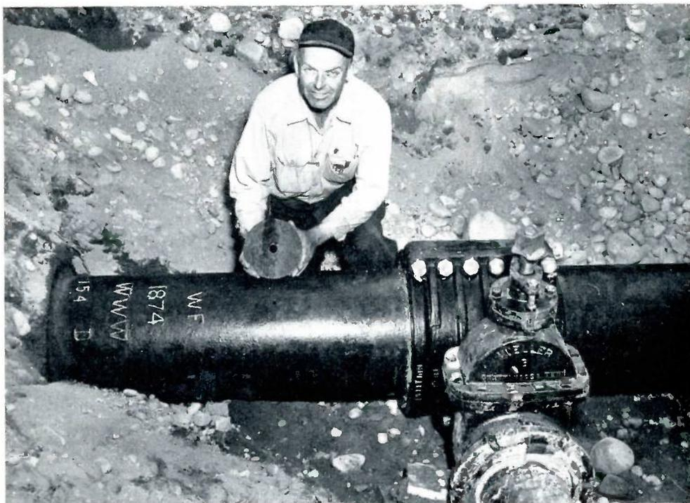
George Brew, foreman, is holding the coupon cut from this 77-year old main. See how clean the cut is. Note, too, that the tapping sleeve fits the old pipe perfectly and that there are no leaks.
