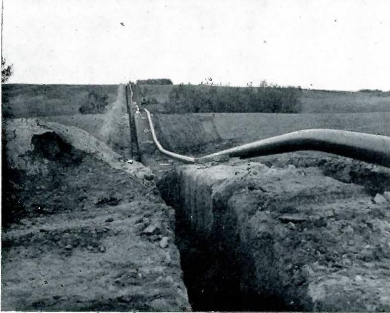
Here is a long section of welded and primed pipe line as it waits the application of protective materials by coating and wrapping crews. Following the wrapping it will be lowered into the ditch and covered with three feet of dirt for adequate frost and farming protection.
