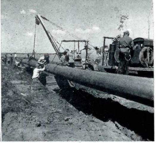
Left: Big rotary machines cutting a trench 5 feet deep and 3 feet wide. Right: Sideboom tractors and welders stringing steel pipe joints along the right-of-way.
