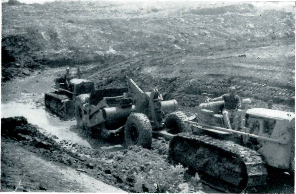
Large earth moving machines digging the lake to desired depth.
