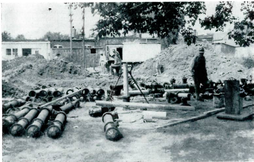
Workmen assemble Mueller Improved Fire Hydrants for installation.
