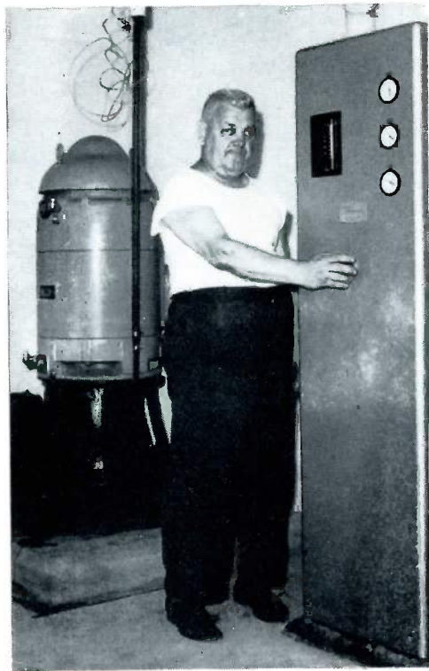
The new one million gallon per day capacity well which was placed in operation in May, 1955. Located in Erskine Park, the operator is S. Rose.
