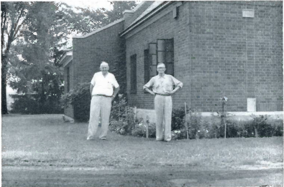
The control building at the South Station which has four wells with a daily capacity of 7,000,000 gallons. Shown are C. Ziegert, left, and F. Hildebrand, operators.
