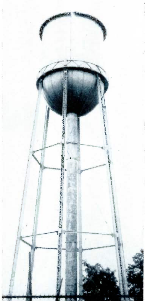
The 250,000 gallon tank at the booster station. Also at the station is a 7,000,000 gallon reservoir. Water is pumped directly from the system to the reservoir. It is then pumped to this tower. Water in the tower rides on the system and is gravity fed into the system.
