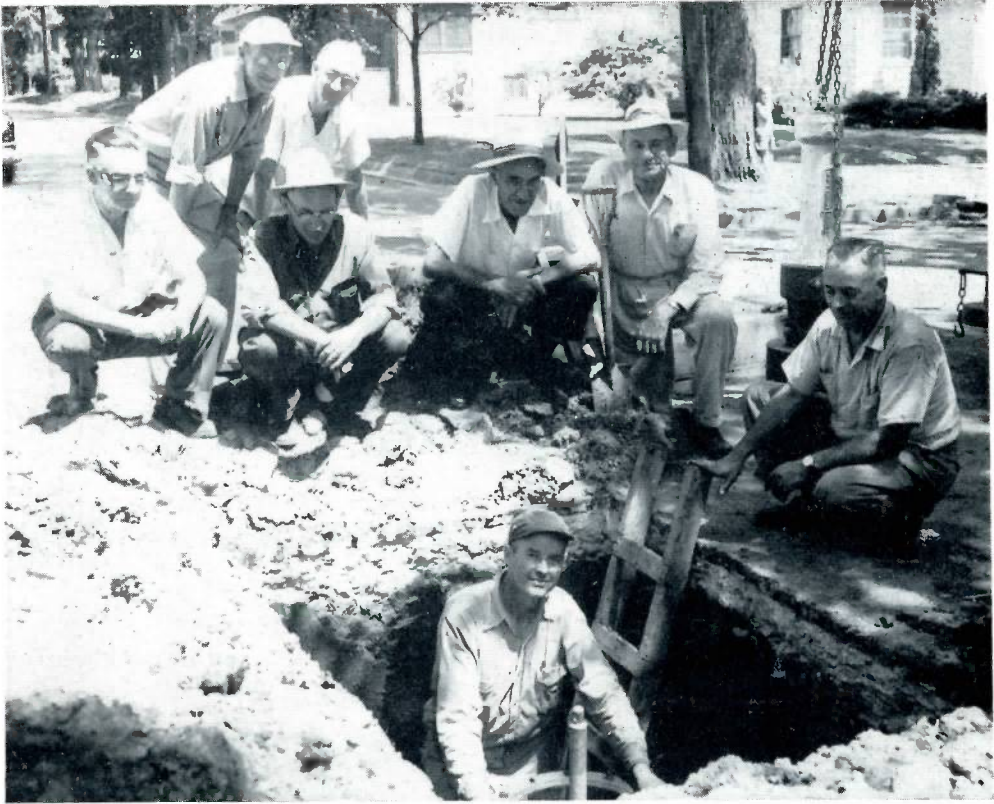
City officials from Oelwein, West Union and Independence, Iowa, crowd around August 4 to watch the installation of a new Mueller inserting valve in a water main on 1st Avenue N. W. Ken Tohill of Boone, Iowa, Mueller sales representative, on the right, checks as M. C. Fangmeier, Waverly City Water Works Superintendent, installs the valve. Watching are Merritt Bushby, Independence city engineer; Grant Bower, West Union Water Works superintendent; Harry Illif, West Union city clerk; Forest Borland and Fred Gremmels, Oelwein city councilmen, and Bill Irwin of the Oelwein Water Works. Top feature of the Mueller valve is the fact it can be inserted without shutting off water along the line. (OELWEIN REGISTER PHOTO.)
