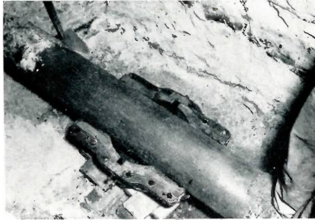
THE FIRST STEP, after readying a main, in installing an inserting valve is leading on the sleeve of the valve, as shown here. This is a six inch inserting valve sleeve on a job in Alpena, Michigan.
