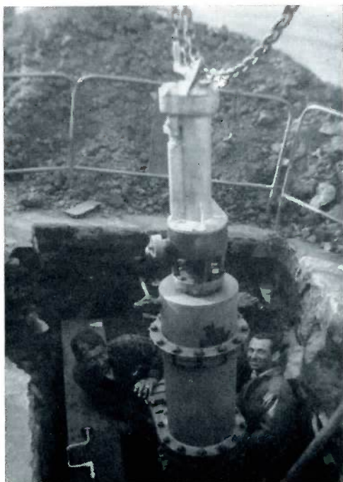
HERE, TWO CLARKSBURG Water Board employees are shown operating a Mueller Valve Inserting Machine. The machine is shown with adapter and 8 inch inserting valve.
