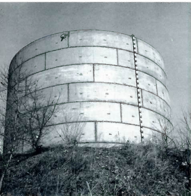
THIS MAMMOTH STORAGE tank is one of two 2,000,000 gallon tanks completed in May for the Clarksburg Water Board.
