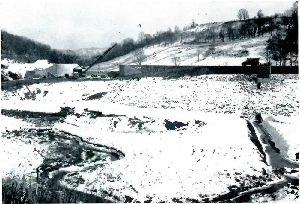
FROM UPSTREAM, the side of the spillway, dam, gate house and impounding reservoir are shown under construction.
