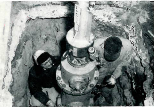
MUELLER CO.'s CC Drilling Machine, with adapter, is mounted on a gate valve to make the cut in the main to put the inserting valve to use. Shown are Mueller Co. Sales Representative Jack Rubicam and Joe Sobeck of the Alpena City Water Department. Working conditions were difficult as the temperature was a cold 50 degrees.
