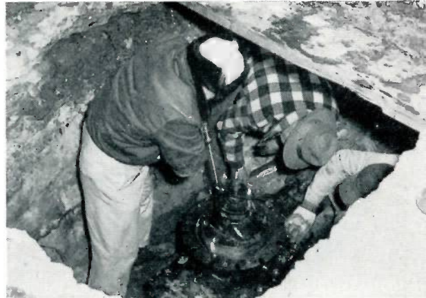
COMPLETING THE installation, the men are shown here tightening the angle packing screws on the inserting valve. Lending a hand is Mr. Rubicam at left. Superintendent of Water, Erling Olsen, is in the center, with Mr. Sobeck at right. The toe of the boot, far right, belongs to Mueller Co. Central Sales Manager Wilson R. Augustine.
