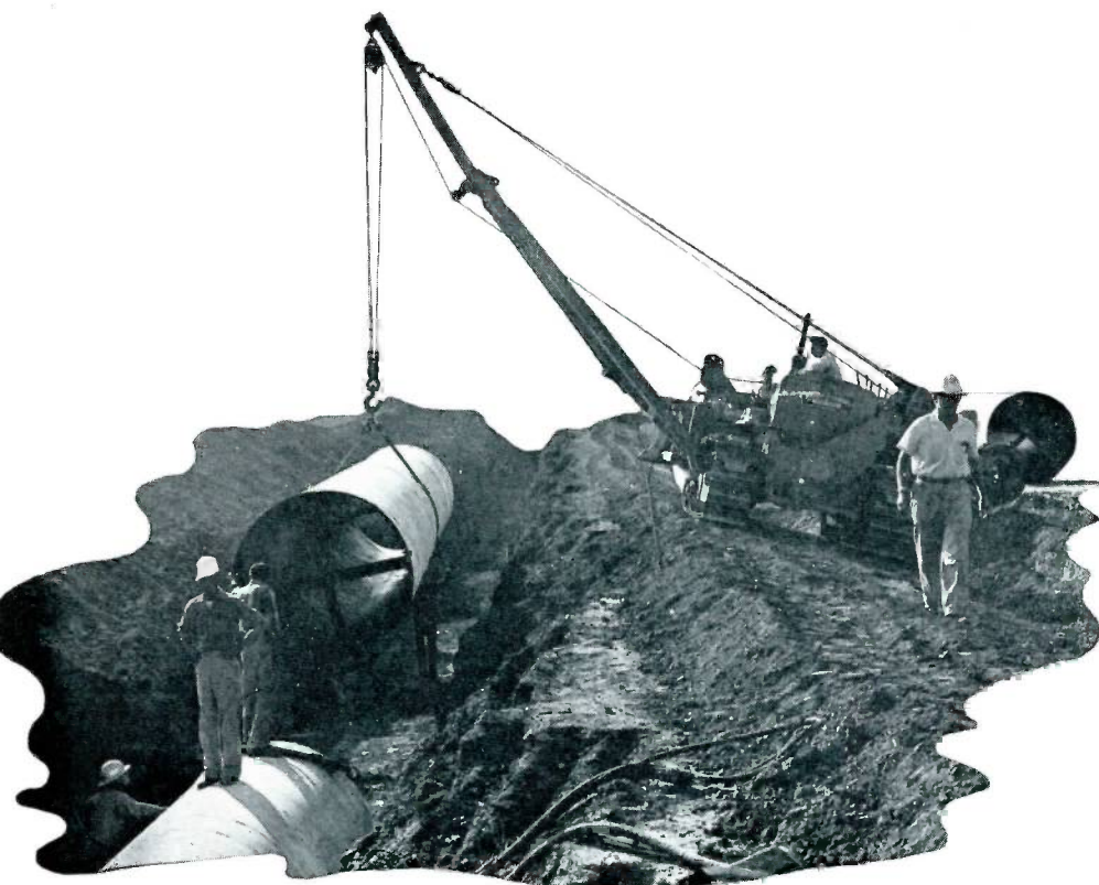
About 24 miles of earth canals, pipelines, checks, discharge lines, siphons and other appurtenances had to be built in the $2,350,000 irrigation project. Nearly two miles of this total were large sizes of steel pipe.
