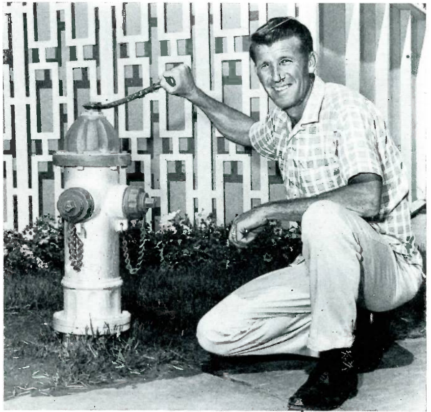
Howard Compton checks a Mueller fire hydrant at Palm City, Calif. Mr. Compton is the city's Construction Superintendent. Below is part of the water plant at Kern City.
