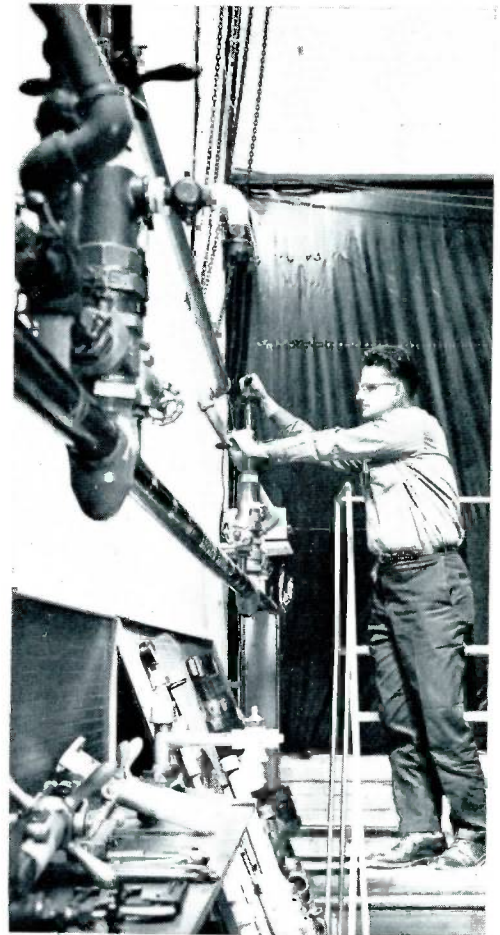
One of the "students" operates some Mueller line stopping equipment on a mock-up line after Mr. Sheerer completed his instruction and demonstration in the lower photo.
