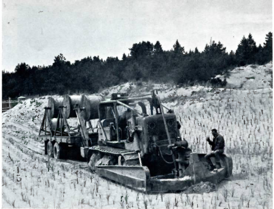
Workmen plow-in power lines for the wells on the dunes.
