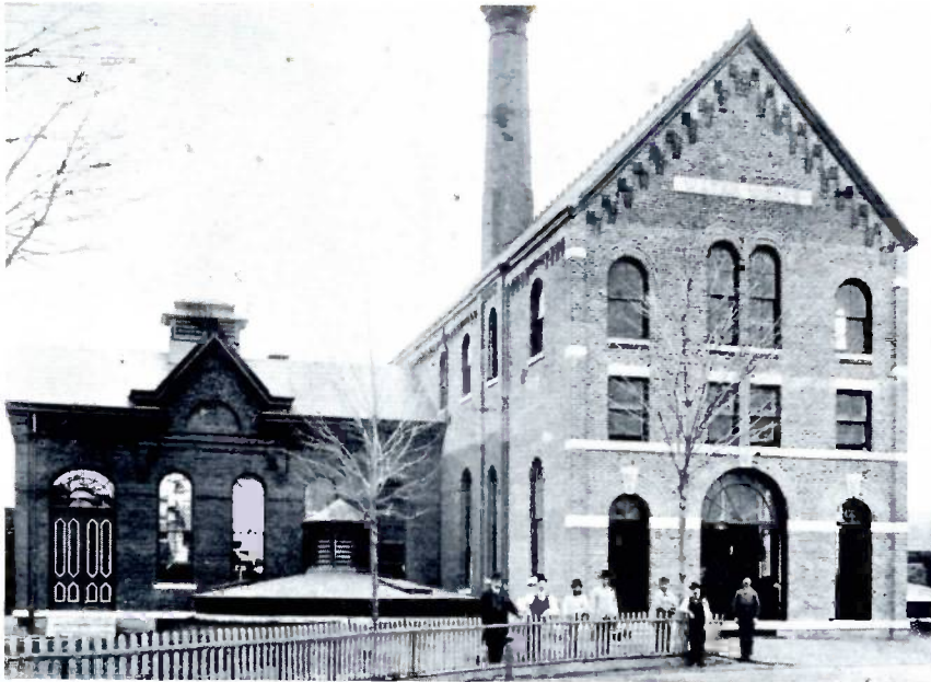
The Binghamton Bureau of Water's original plant was built in 1867 and put in operation a year later. It took water directly from the Susquehanna River and pumped it directly into the mains.
