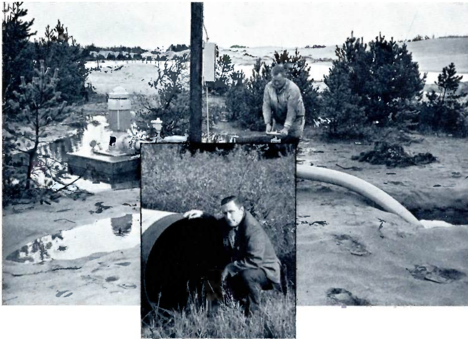
General Manager-Chief Engineer C. W. Heckard (inset) inspects a 38-inch pipe which will be part of the collector pipeline between the wells on the dunes. Dunes Water Source Operator Bernard Finell checks a valve on well #49, delivering 220 gpm to a local industry.
