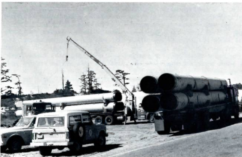
This 38-inch pipe is used as part of the collector system for the wells on the dunes.
