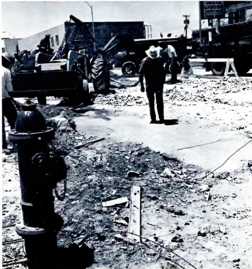
Tractors and trucks were the traffic on the main street in Denison for many months during the construction of the Denison "Shopping Park." Mueller Hydrants seemed to be located in the middle of the street, but the winding driving lanes returned the hydrants to their proper place when work was finished.
