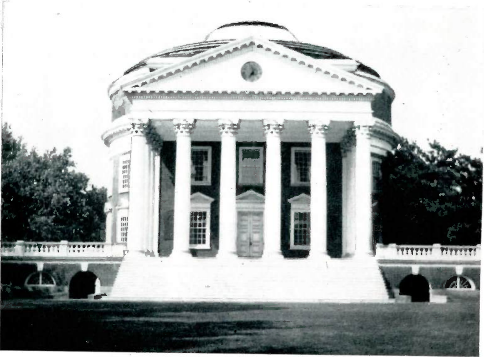
The water tank was located in the top of the famous Rotunda building of the University of Virginia. It has since been removed.
