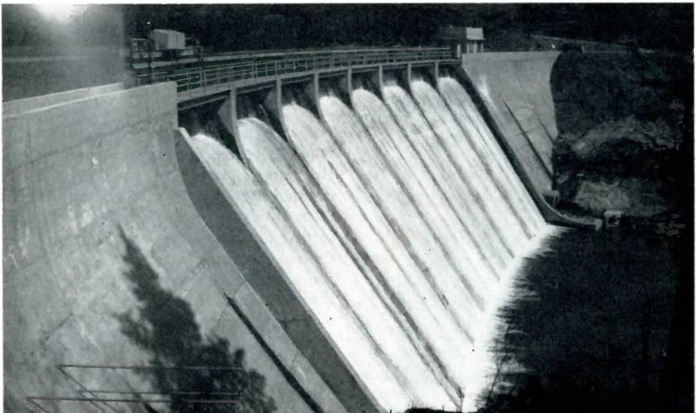
View of the Moorman's River dam.
