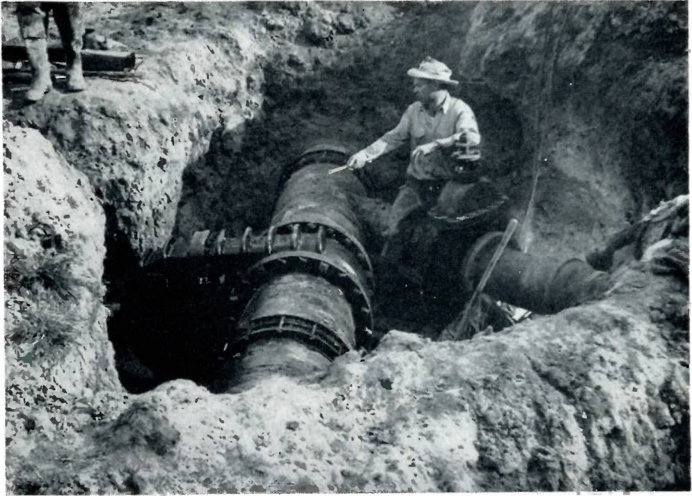
This 24-inch Mueller gate valve was one of many Mueller Co. products installed by the California Water & Telephone Co. during its expansion program.
