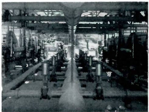
This is an inside view of the filter plant showing a few of the big filter units and a portion of the network of pipes, valves and gauges.
