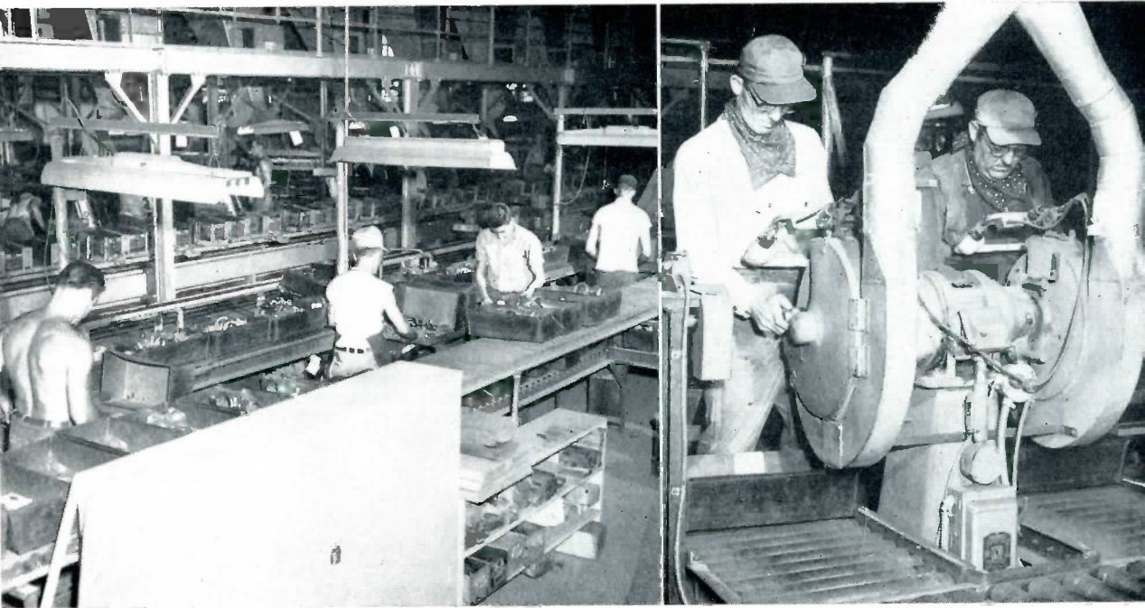
Castings are sent through a cleaning process which removes adhering sand and cores, and gives them a golden bronze appearance for which our products are well known. They are sorted, placed in pans and then travel on a conveyor to the four men at left who inspect them and remove any with visible defects. Once inspected, castings continue their journey to the grinders where gates and fins are removed. Two grinders are shown at right.
