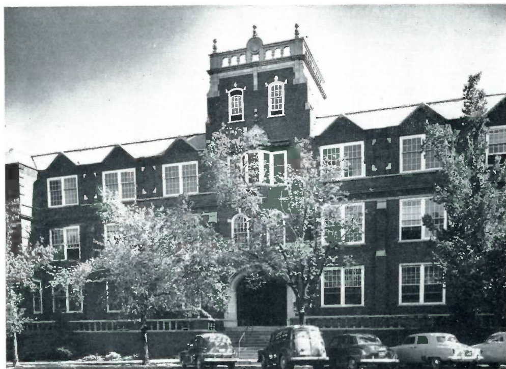
The Administration Building at Stephens College in Columbia.
