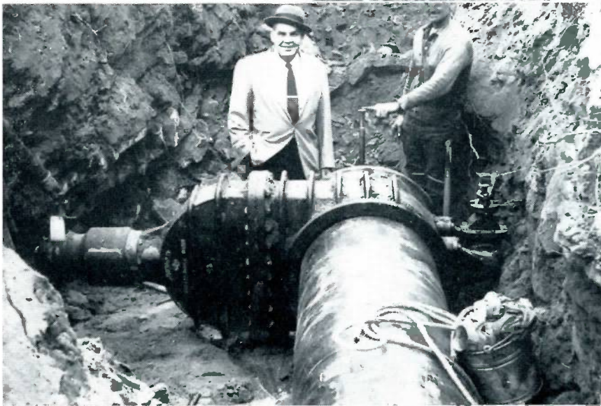
To the left and below, Mr. Don Calderwood, president of Pennichuck Water Works, stands beside a Mueller 24-inch valve which has just been completed on the line.
