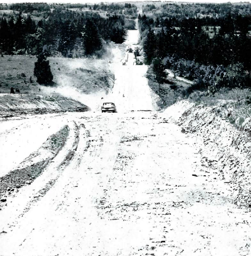
Clearing Tolt River pipeline right-of-way in preparation for laying pipe. A maintenance road will also occupy this right-of-way.
