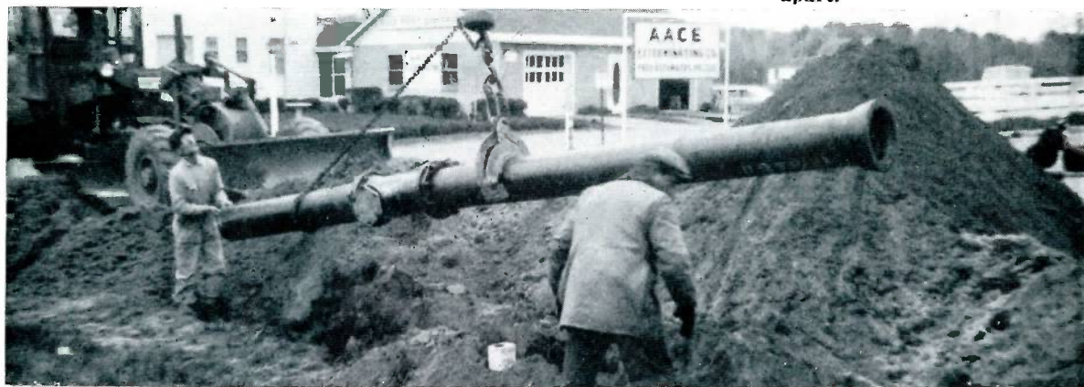
Standard pipe tongs are one of the three basic tools used in the extensions of water mains for this New York utility. Workmen are shown maneuvering a
