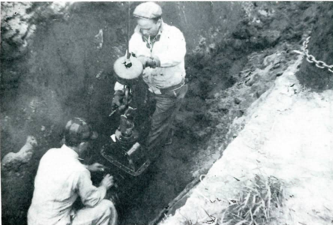
A 10-inch Mueller gate valve is set in place with little lifting by workmen (left). The tool slips over the crane hook and under the operating nut on the valve (above). The lip of the tool is built up so that the valve can't slip off.
