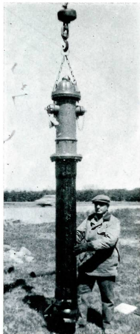
One of the devices used by the City of Saratoga Springs for lifting Mueller Improved fire hydrants is shown above. This is installed by removing two bonnet bolts 180 degrees apart.
