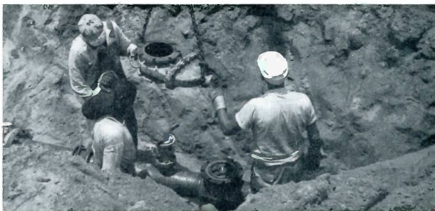
After the tee and valve are coupled in place (left), the line stopping unit was removed and the completion machine used to insert the completion plug shown above. The gate valve is being removed so that the cap can be put on the fitting.
