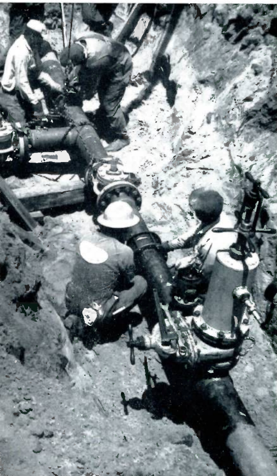
After the tee and valve are coupled in place (left), the line stopping unit was removed and the completion machine used to insert the completion plug shown above. The gate valve is being removed so that the cap can be put on the fitting.
