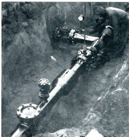
With the cap in place (right), the job is nearing completion as a workman applies a coating to the new installation. Savannah Gas Company's Robert Smith, a project engineer (below), checks the site for a water crossing.
