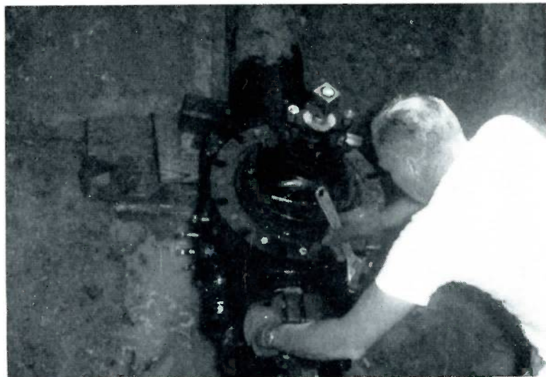
The two-part sleeve is installed around the main in the photo above, while the photo below shows the same sleeve after the valve body has been installed and about ready for use.
