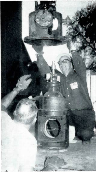
Mueller Sales Representative Ken Tohill guides an adapter over a valve body as work continues to insert a new gate valve into an existing water main that remains under pressure.
