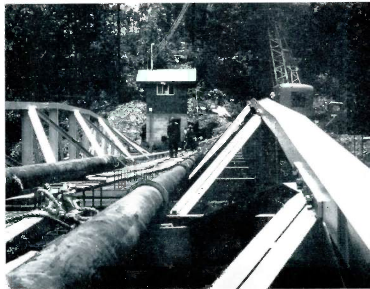
Two, eight-inch lines carry the lake water from the barge to the control house where they merge into a single line leading to Dadeville's filter plant.
