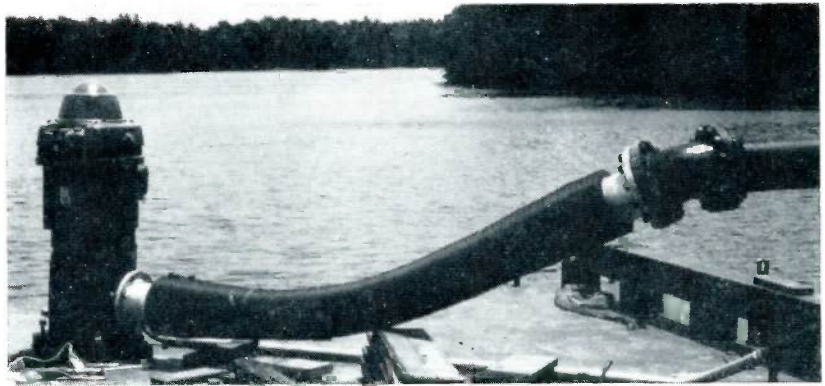
This 10-foot long piece of hose provides the flexibility that is necessary between the rigid pipe and pump. Each Byron-Jackson pump is capable of pumping 500 gallons per minute.
