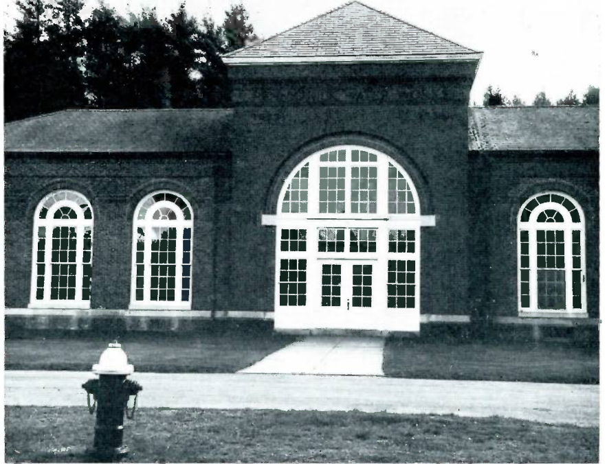
The left wing of Snow Pumping Station houses diesel pumping units which have a capacity of 5.8 MGD. The other wing contains two electric-powered pumping units which have a combined capacity of more than 13 MGD.
