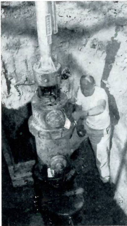
This Mueller drilling machine is used to lower the valve body through the long and short adapters into the valve sleeve. In an earlier operation, the drilling machine was used to make the cut in the main.
