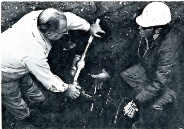
It isn't unusual to find a Mueller sales representative in the ditch talking to the men who use our equipment or giving a hint on the proper installation of Mueller products.
