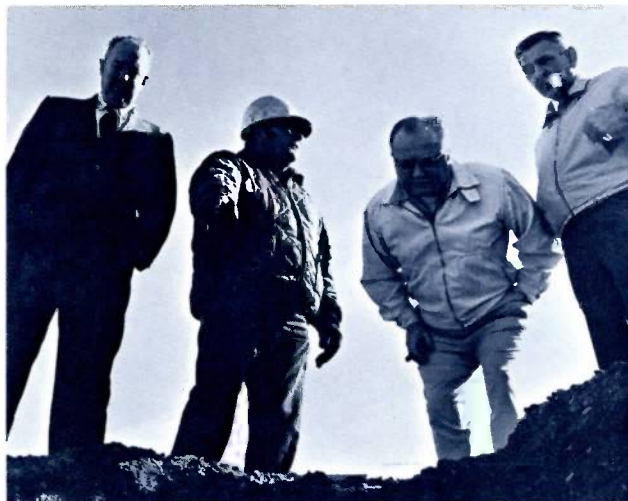
A construction foreman in Waukesha points out an operation to Jack, Joseph Kuranz, left and Clayton Brimmer, right. Mr. Kuranz is manager of the Waukesha Water Department and Mr. Brimmer is superintendent of construction.
