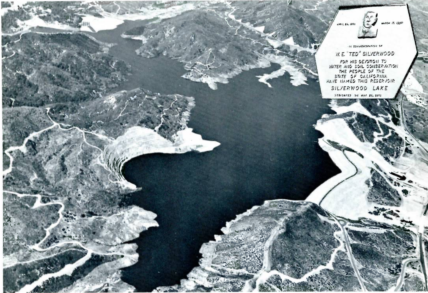
Silverwood Lake, behind Cedar Springs Dam, is an important facility in the California State Water Project. The inset shows a plaque honoring W. E. "Ted" Silverwood, a California conservationist after whom the lake is named.
