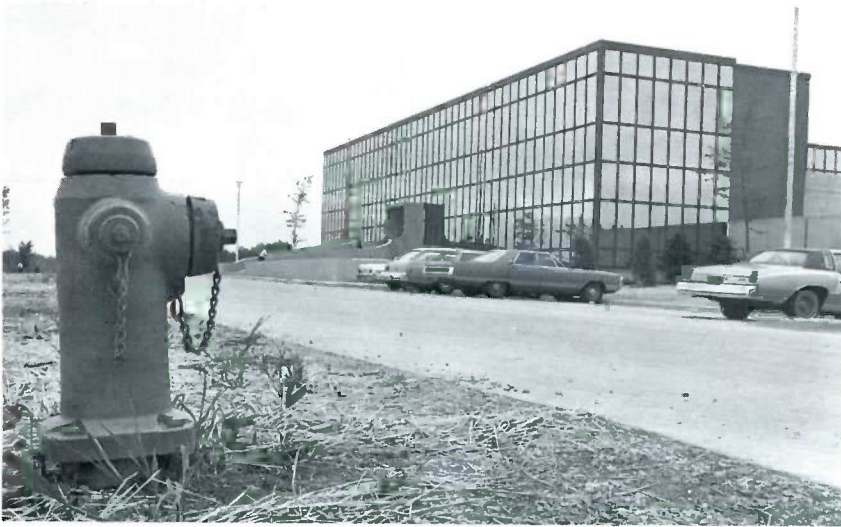
In the foreground a MUELLER Modern Improved Fire Hydrant. In the background the North Water Treatment Plant.
