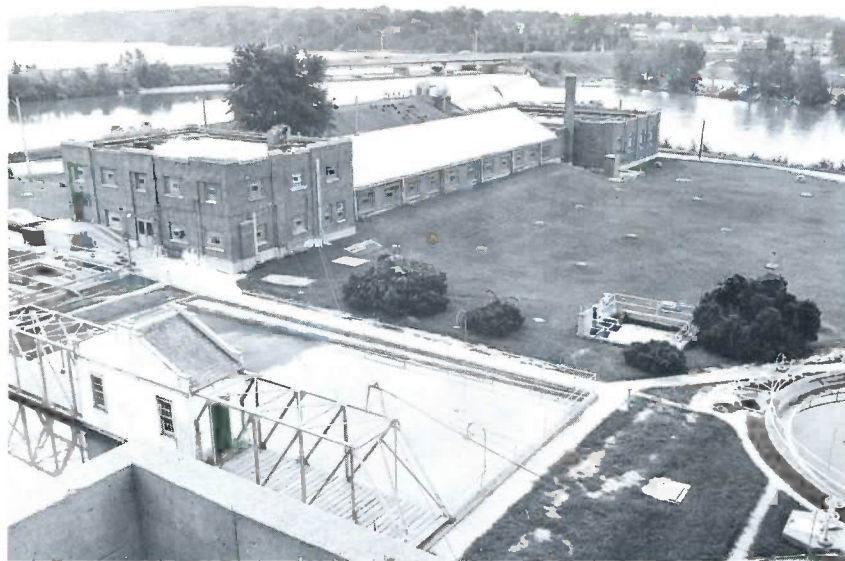
Original water treatment plant with dam and Lake Decatur in background.
