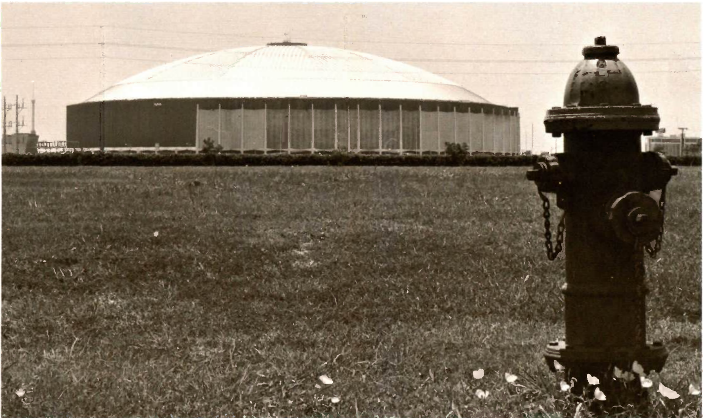
Mueller fire hydrants also stand guard around the famous Houston Astrodome. This mammoth, air-conditioned, convertible structure is home to the Astros, the Oilers, the University of Houston athletic teams, as well as the site for rodeo, track and motorcycle races. Billy Graham, Evangelist, has dubbed it "The Eighth Wonder of the World."
