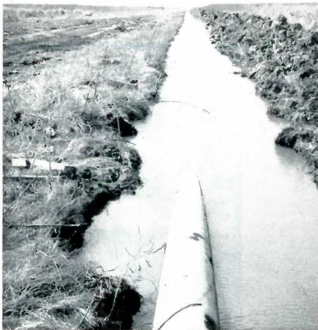
The 16-inch pipe was welded together, section by section, and shoved down the ditch by "cats."
