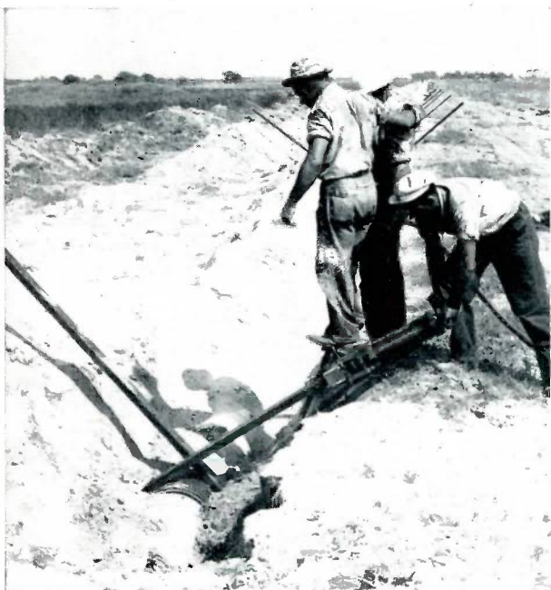
Two ten-foot lengths of four-inch channel iron serve as a huge fork to pin the pipe in place. These anchors are slipped through grooves in cushioned pipe saddles and are driven down with an air hammer.
