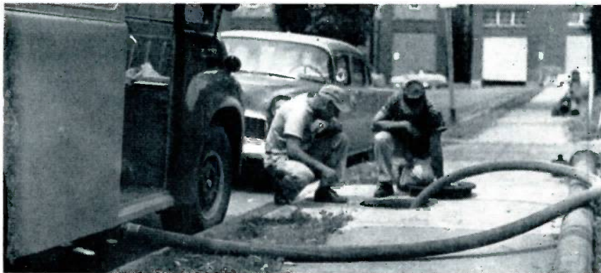
Left: Testing a meter in the field with the Water Meter Maintenance Truck. A hose is connected to the meter, which is encased in a vault, and the hose leads to the calibrating equipment within the truck.
