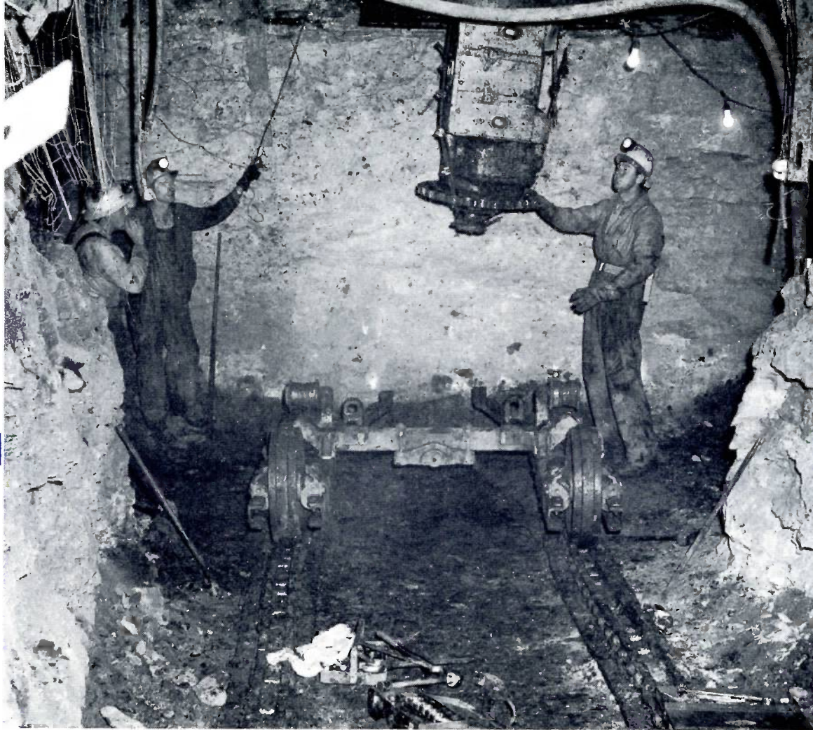
As the mined area extended farther from the shaft, heavy big tractors were lowered piece-by-piece into the cavern. The motor of the tractor can be seen just as it emerges from the end of the shaft.
