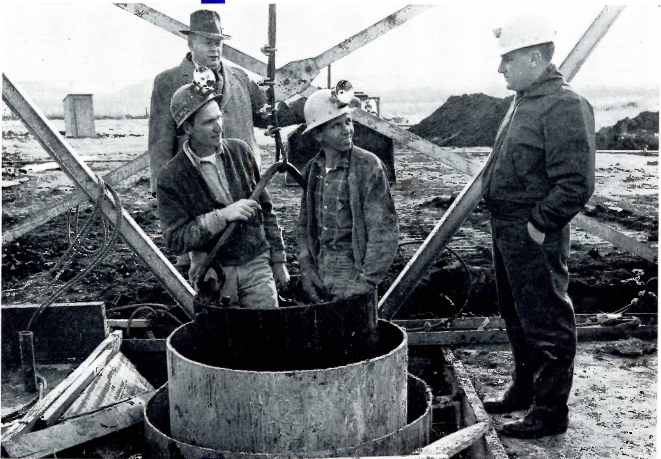
Buckets are also used to take workmen back and forth from the surface to the work area. When the mining operation began one or two men started digging by hand and as the cavern grew in size larger crews were needed. The mining was carried on 24 hours a day, six days a week.
