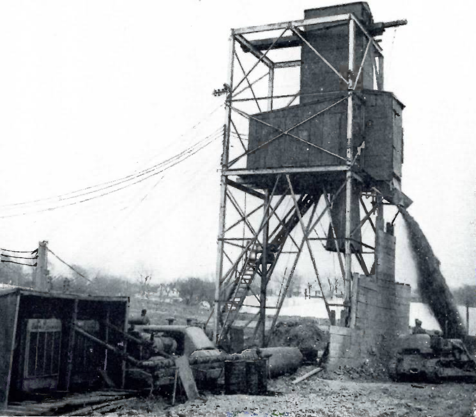
A tippel was constructed over the shaft with the enclosed portion housing the hoisting equipment. During peak mining, buckets filled with material were raised to the surface and dumped every 40 to 50 seconds.
