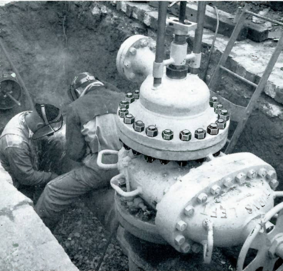
6. Once the shut-off is made workmen are free to proceed with their work. They have cut out a section of the isolated pipe (above) and safely are able to weld (below).
