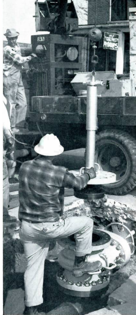
7. Once the work is complete, the stopper is contracted and removed, and the gate valve is closed again. The next step is to install the completion plug in the fitting (above), and remove the completion machine and valve.
