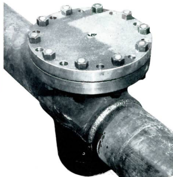
7. Once the work is complete, the stopper is contracted and removed, and the gate valve is closed again. The next step is to install the completion plug in the fitting (above), and remove the completion machine and valve.
