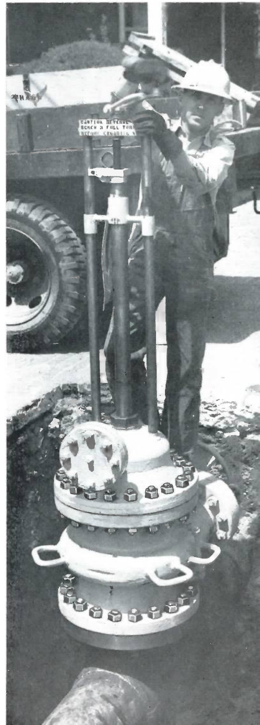
5. Workmen here are attaching the steel wedge stopper to the machine prior to bolting it to the valve. Once it is tightly bolted to the valve, the gate valve can be opened and the stopper lowered into the pipe through the two holes made by the drilling machine. After it is in the fitting and the pipe, the stopper is expanded (lower right) and the shut-off is made.
