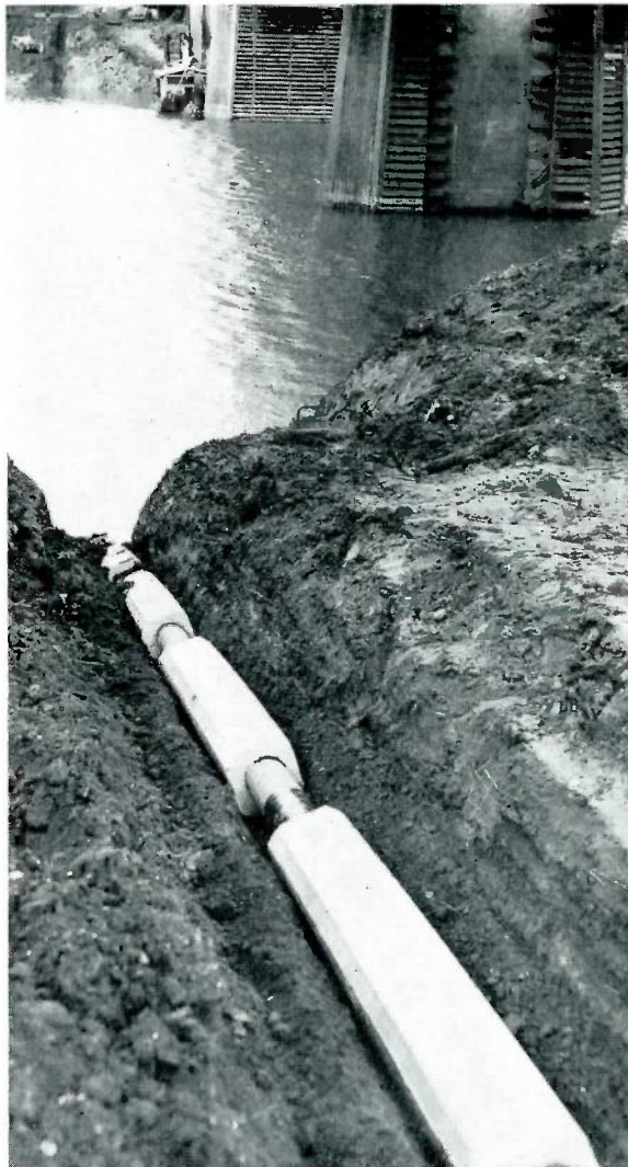
Heavy concrete weights are put on the line so that it will rest on the river bottom without moving with the currents.
