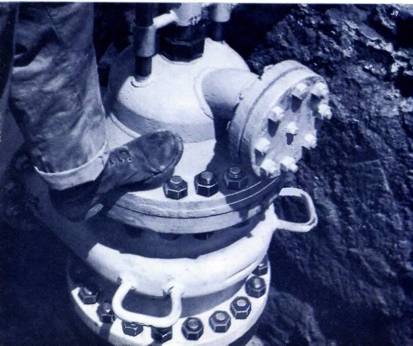
4. After the cut is complete the cutter is withdrawn to the rear-most position and the gate valve is closed so that no gas will leak into the atmosphere. The machine is then removed and blocked (above) so the steel cutting tips are not dulled by scraping on the pavement. Below is a close-up shot of the line stopper in position.
