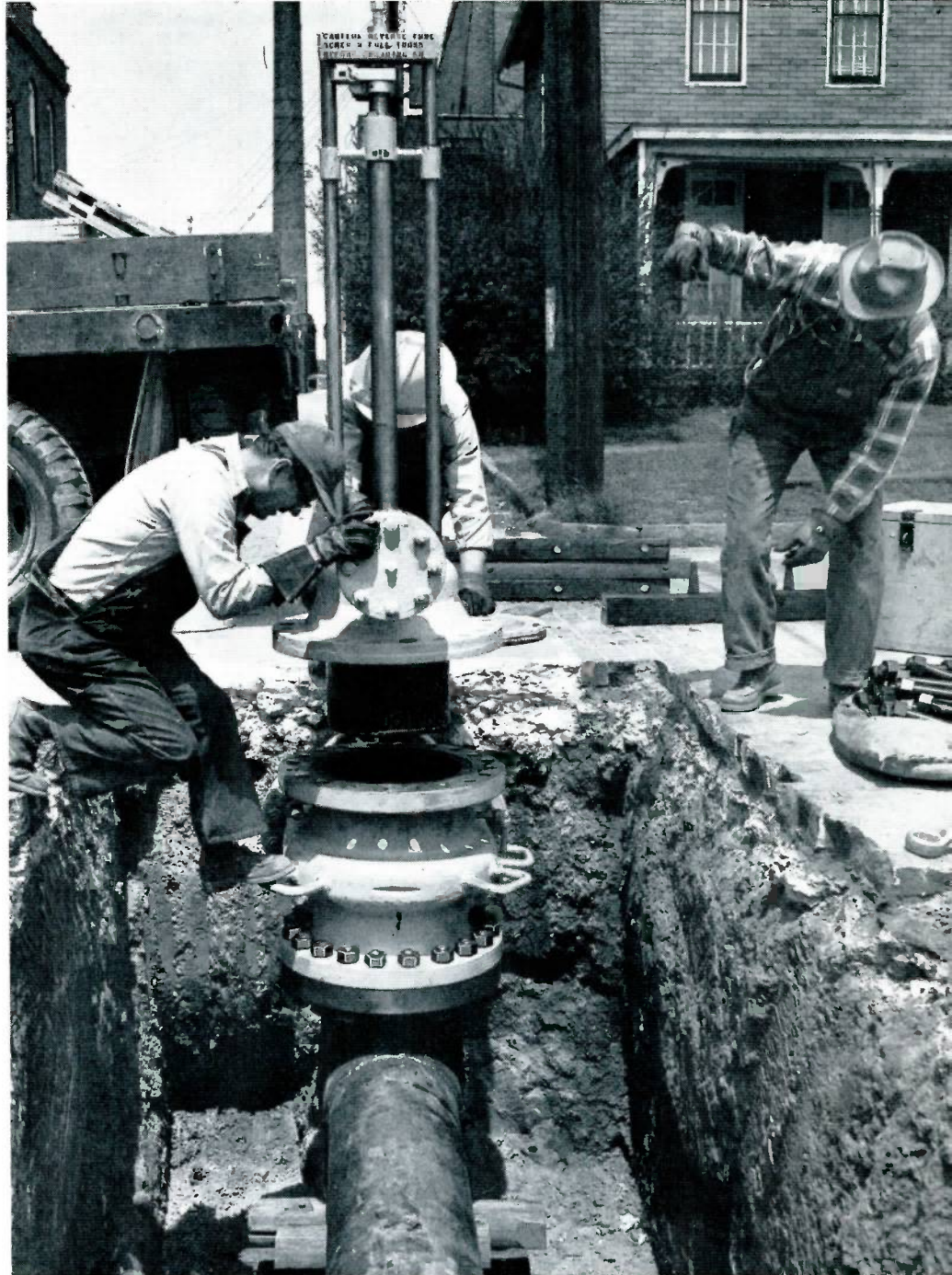
Illinois Power Co. workmen lower a Mueller 4SW Line Stopping Machine into position preparatory to isolating a section of a 12-inch gas main. The following picture story tells how Mueller No-Blo fittings and equipment accomplished this task.
