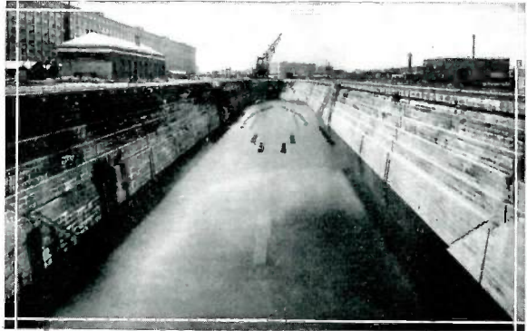
Drydock Boston, Mass. Largest drydock on the continent and the only one in America large enough to accommodate the S. S. Leviathan which comes to Boston for overhauling. The dock was built by the Commonwealth of Massachusetts and completed in 1919. In 1920 it was sold to the Navy for $4,158,385. It is 1,175 feet long, 149 feet wide, and 44 feet nine and one-half inches deep. —Courtesy of the Boston Chamber of Commerce.
