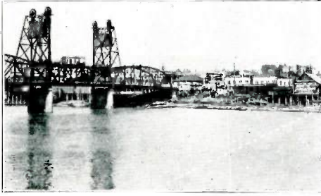
Bridge across Cowlitz river which separates Longview and Kelso showing the location of the main laid 16 feet under the bed of the river to serve the two cities from the manufacturing plant in Longview.
