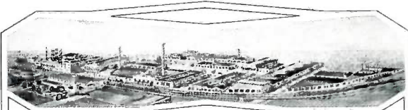
MAIN PLANT Decatur, Ill.
