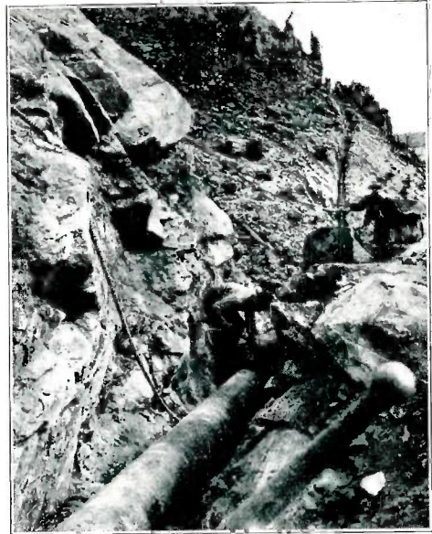
Cutting a 16" O.D. Matheson Joint pipe, National Coating, with air hammer, in Yankee Doodle Canyon, for installation of a fitting. Joints caulked with air hammer under 140 pounds maximum pressure. Miles of mains of the Butte Water Company are imbedded in solid rock. This scene is typical of the engineering and construction problems which Mr. Carroll battled with successfully.
