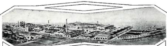
MAIN PLANT Decatur, Ill.
