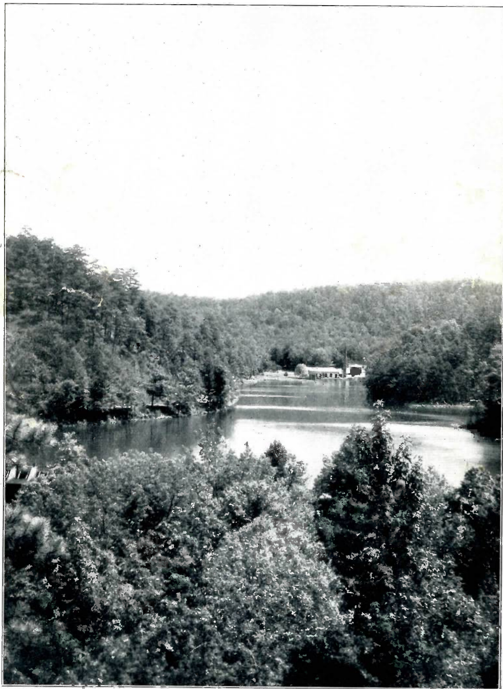
BEAUTIFUL SETTING OF HOT SPRINGS, ARK. PUMPING PLANT
