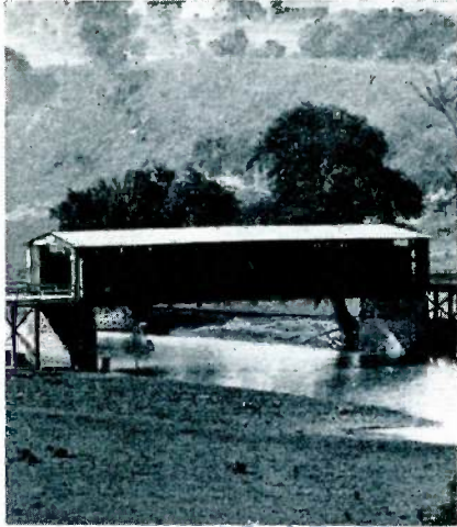
Macon County's Last Covered Bridge
