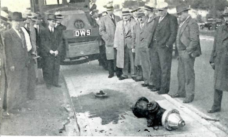
New York officials see big truck breaking down Columbian hydrant under pressure.
