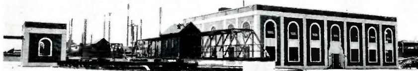
Louis P. Booz, Construction Engineer, Designer of Sewage Treatment plant at Perth Amboy, New Jersey's Chemical Mechanical System. Above — Interior View of Sewage Treatment plant. Below — General View of plant.
