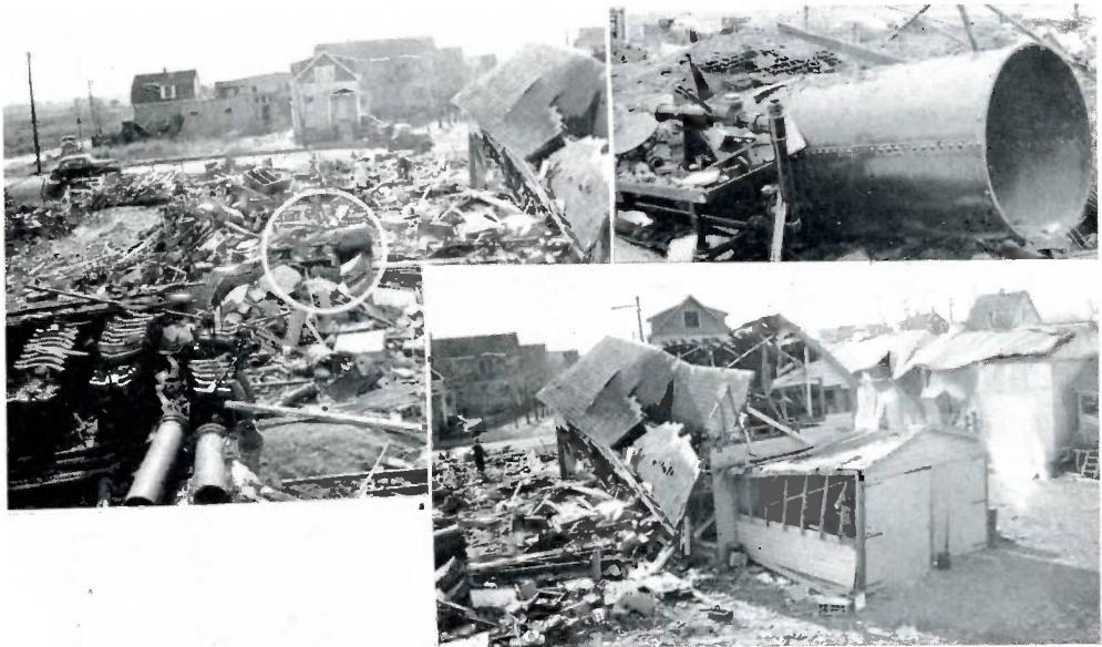
Left: In circle is shown a Mueller Water Meter Tester in midst of debris. Upper right is a close up of the Mueller Tester and Tank. Lower right: What was left of the store house and meter shop.
