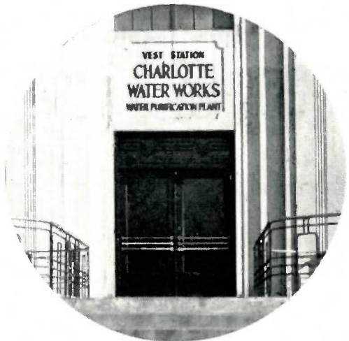
Entrance to Vest Station, Charlotte's 17-million-gallon-per-day filtration plant, which was named in honor of W. E. Vest, the city's veteran consultant and former superintendent.
