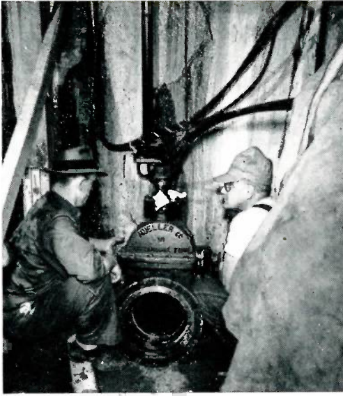
Chepan and Ehram look over the installation of the tapping sleeve and valve on the 10-inch steel line from the clear well.
