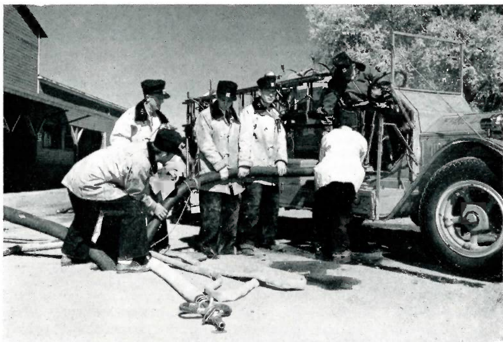
Next step is connecting up the intake hose to the pumper. Here the firemen are connecting up No. 1 truck. The intake hose to No. 2 truck already has been connected. The firemen here are Sanderson, Crinklaw, Riley Masseger, Chief Howard, Harold Ferguson and Williams.
