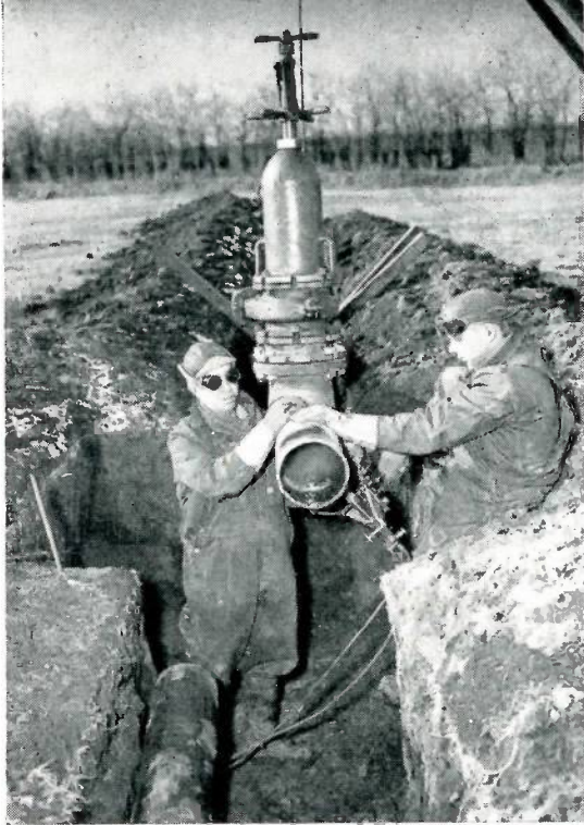
The new line just misses being a perfect fit, and Shacklet and Riggs pare off a small section of pipe with an oxy-acetylene cutting torch.
