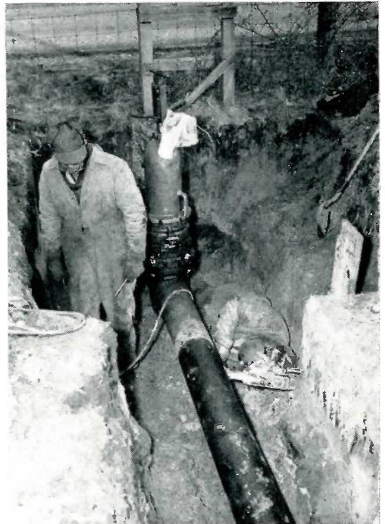
Welding the line on the upstream side of the station completes the by-pass and ties on the Shell Oil Company's new pumping station.
