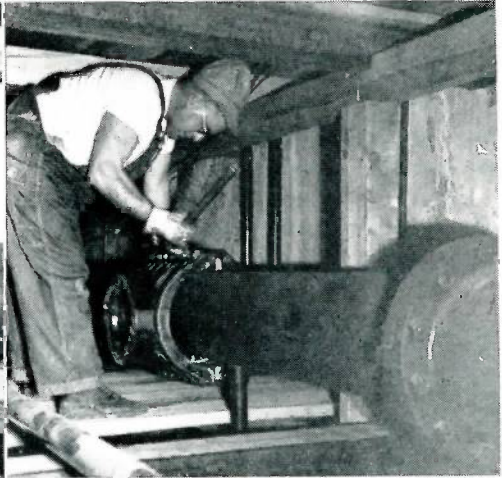
Roy Ehram, water works employee, bolts on the 12" by 8" tapping sleeve before it is calked and leaded to the 12-inch steel feeder line to the city.
