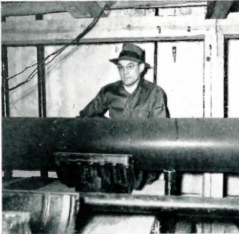
Jack Chepan, Mueller Co. service foreman, is shown with half of the tapping sleeve at the point where the main feeder line, under 125 pounds pressure, was cut.
