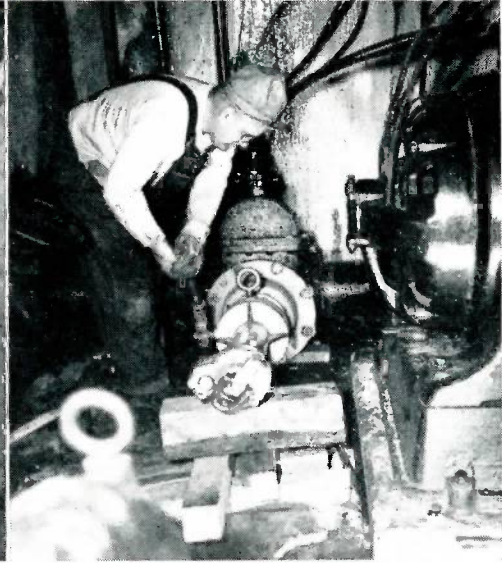
Ehram operates the Mueller C-C machine as it completes the 10-inch cut in the clear well line. The cramped quarters are apparent.
