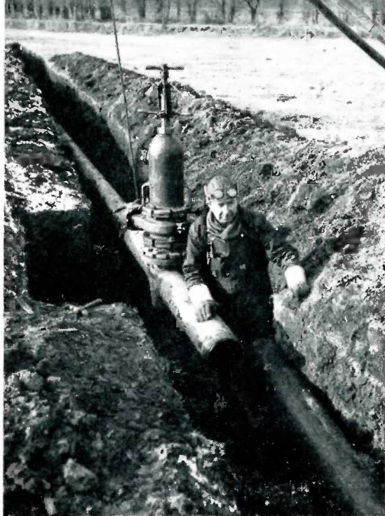
A new section of line, by-passing the old station, has been laid in the ditch. Welder Howard Shacklet watches as the crew trues up the line.
