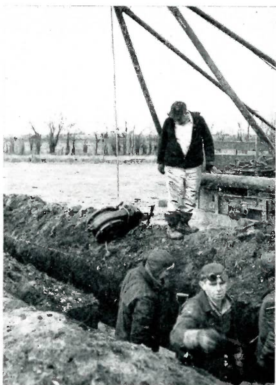
The completion plug has been inserted in the welding fitting, and the gate valve is lifted out of the ditch to permit permanent tightening.
