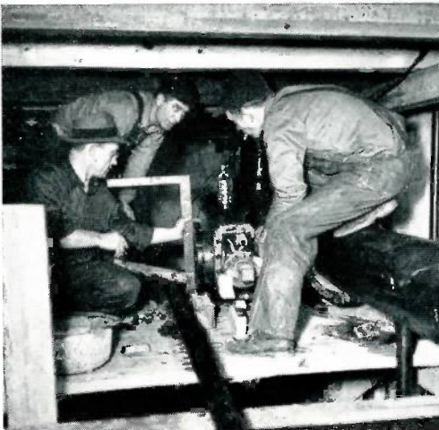
Chepan checks valve's alignment with Glen Wilson and Marion Myers, Charleston water works employees.
