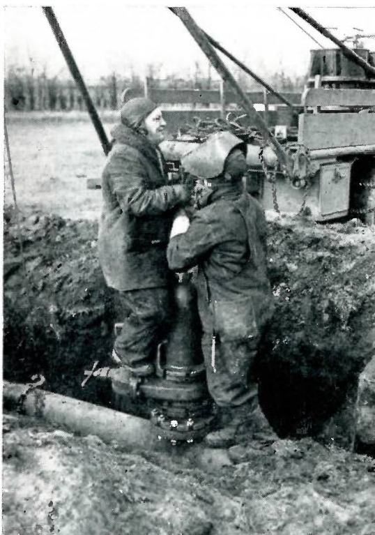
Welders Art Reed and Shacklet apply a little heave-ho to withdraw the stopper. The H-17335 stopping machine is then unbolted and removed.
