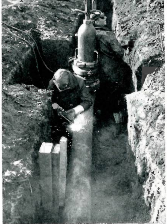
Welder Shacklet then joins the new section to the main pipe line with an electric weld, and the down-stream by-pass is nearly completed.
