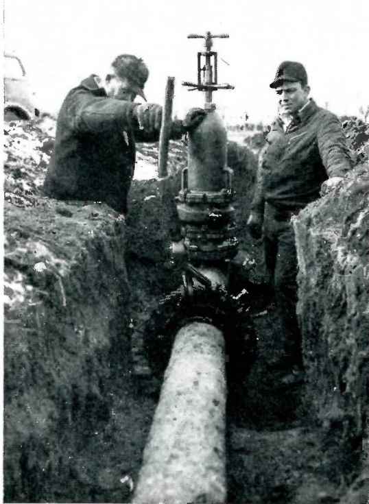
Next step is the actual cutting of the pipe line. Maintenance Foreman O. H. Day, left, checks the alignment of the cutter before the line is severed.
