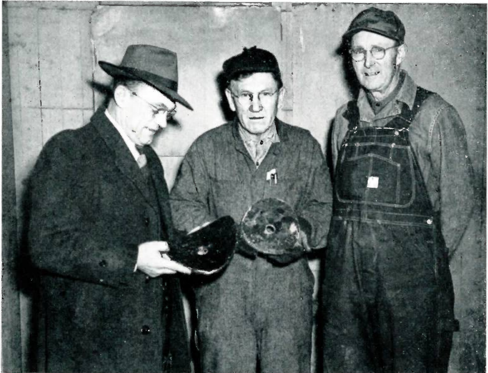
The job completed, Chepan holds the 10-inch steel coupon cut from the clear well line and Ervin Light, center, water superintendent, is shown with the 8-inch coupon from the main feeder line. Henry Elliott, water works employee, is on the right.
