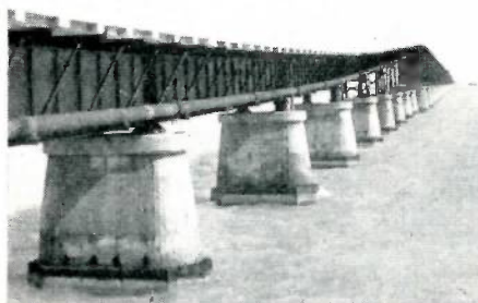
The pipe line makes an over water crossing along a bridge of the Overseas Highway on its way to Key West.
