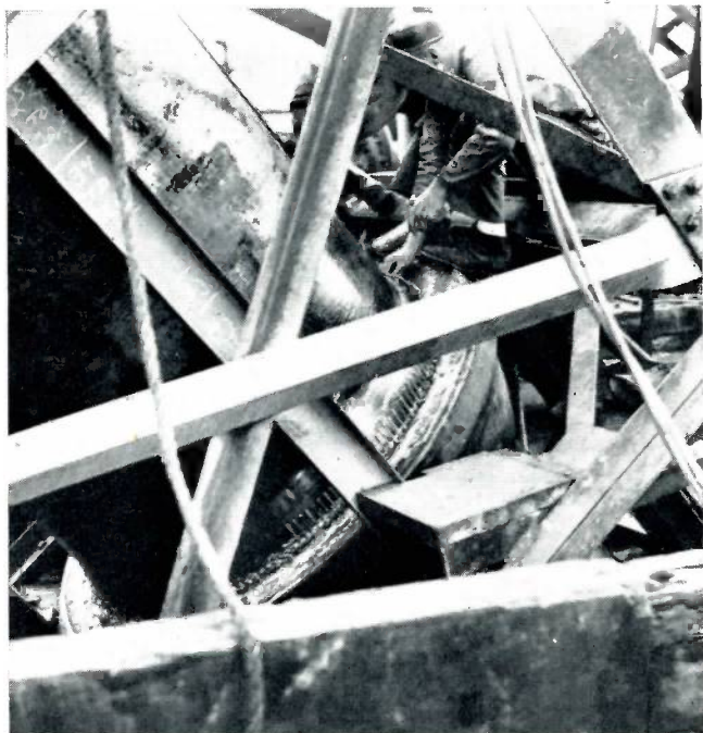
Flexible joint with bottom third nailed and caulked, and nails set in top two-thirds.
