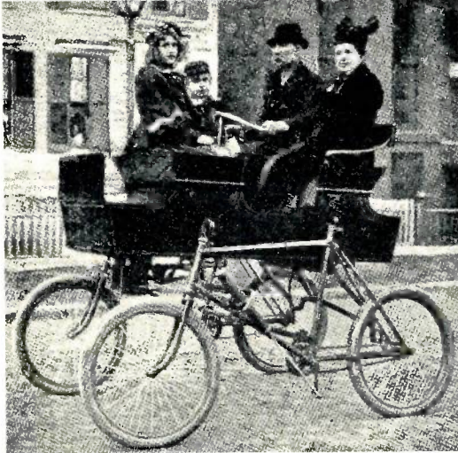
The A. C. Ames car, having a two-bicycle chassis and a sleigh body, was steam powered. The car was "steamed up" at Chicago and ran a few hundred feet indoors, thus qualifying as operative.
