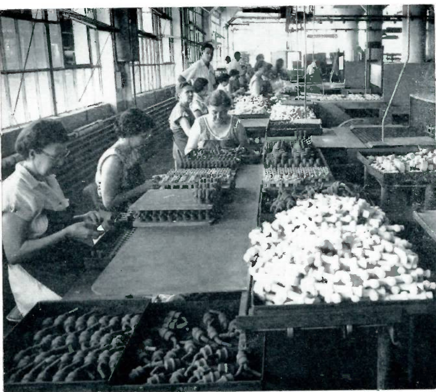
Baked cores are cleaned and inspected by our large staff of Core Room inspectors before being conveyed to the core storage area.
