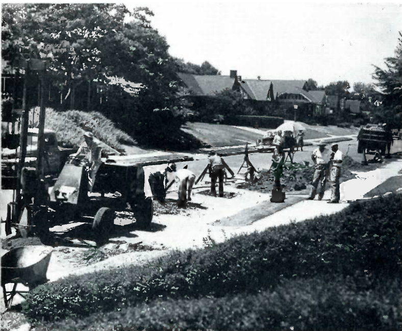
This photo shows a crew installing a coated and wrapped 22-inch pipe for an orifice meter at the Weaver Road Station.
