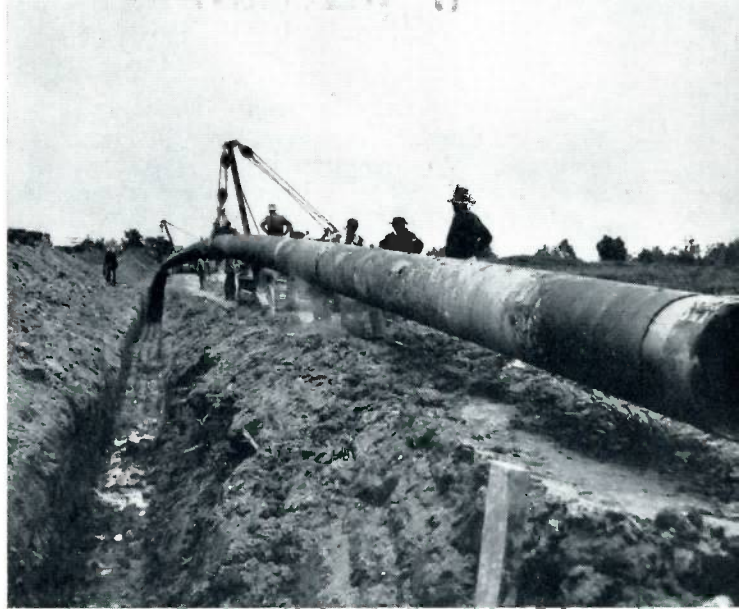
This crew is lowering a coated and wrapped 22-inch pipe into a new trench. The pipe was designed for 500 psi.
