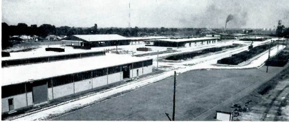
This is a view of the new Gas Service Center of the Memphis Light, Gas and Water Division. When construction is completed in 1958, it will be among the finest such installations in the country. The buildings are housed on a 44-acre section, and a modern pipe-coating and wrapping plant was built in 1953.
