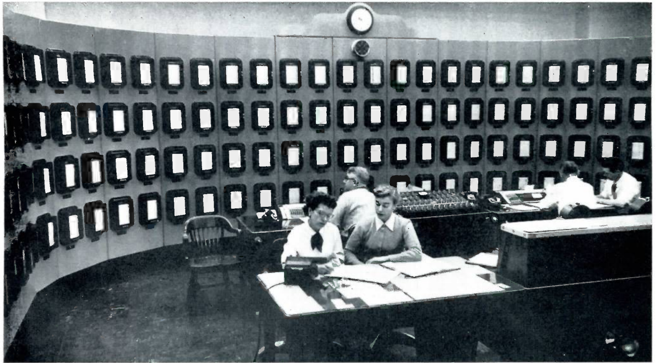
The Gas Dispatcher's Office is a busy and efficient place. This is a partial view showing some of the 198 teletyping devices in operation. In addition, there are 72 district pressure regulators remotely-controlled from this office.
