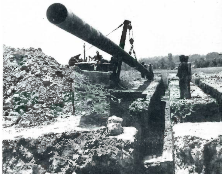
This photo shows a crew installing a coated and wrapped 22-inch pipe for an orifice meter at the Weaver Road Station.
