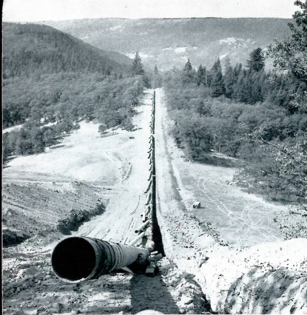
This is a view of the Corning-Eureka gas line on the west side of South Fork Mountain between Dinsmore and Summit, California.
