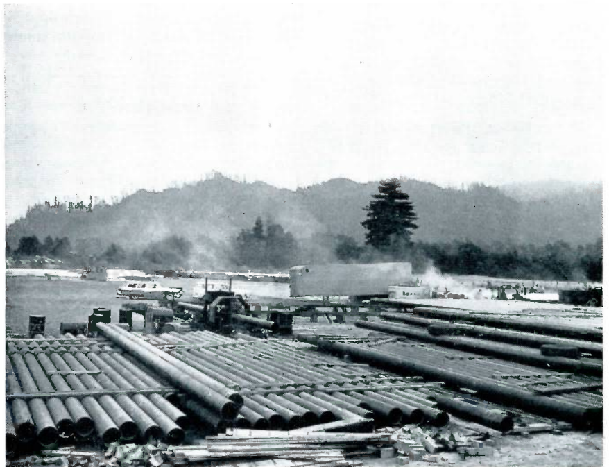
The pipe camp discloses lengths of pipe ready for use in PG&E's new gas line.
