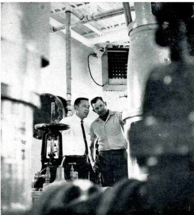
Supt. Kindel gives Mayor Hahn a tour of Booster Station No. 2 which recently went into service as part of a new automatic system.
